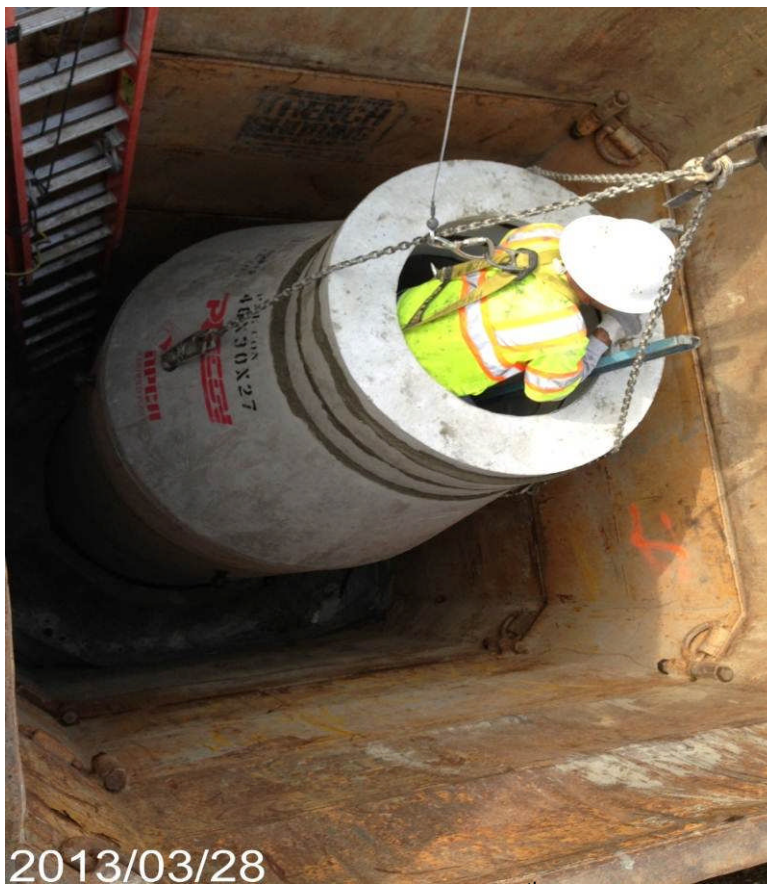
Advanced Utility Relocations contractor at 60 th Street seating of manhole.
