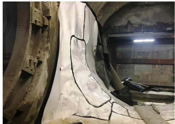
HDPE Application at Reach 1 Cross Passage #11
