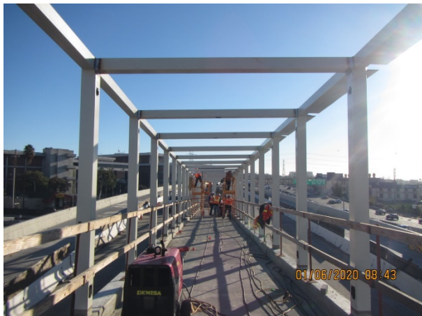
Pedestrian Bridge: Erecting structural steel
