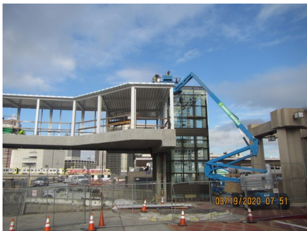
Installation of elevator outside glass
