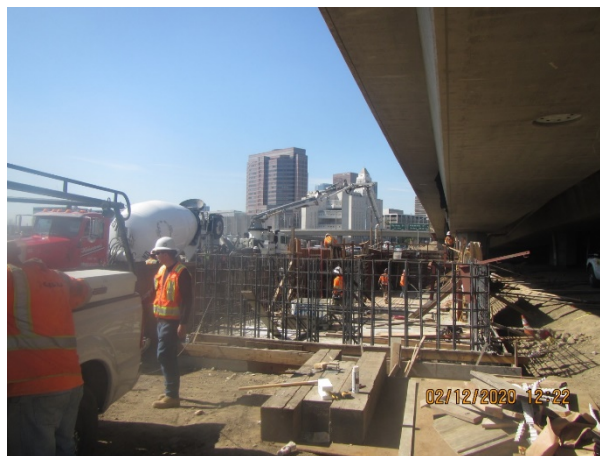
Austin Vault: Rebar installation and pouring concrete
