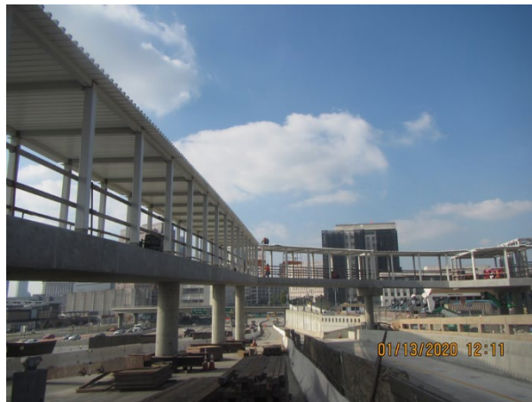
Installation of metal roof deck
