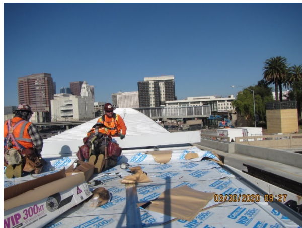
Installation of Pedestrian Walkway roof
