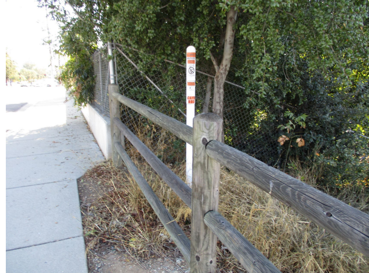
Fencing Upgrades (Prevent Trespassing and Accidents)
