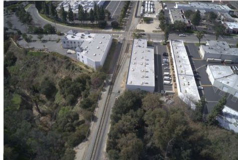
Deep Ravine Arch Brick Culvert
