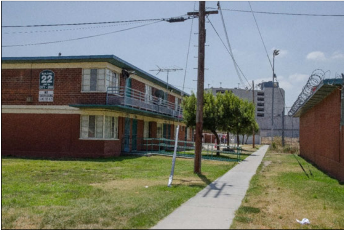
Figure 5-11. Key View #1b – Existing Condition (Retaining Wall)
