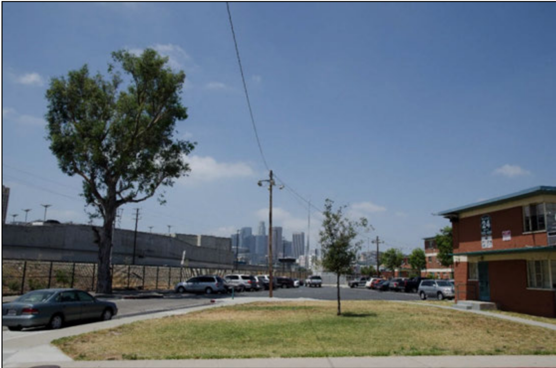
Figure 5-9. Key View #1a – Existing Condition (Retaining Wall)
