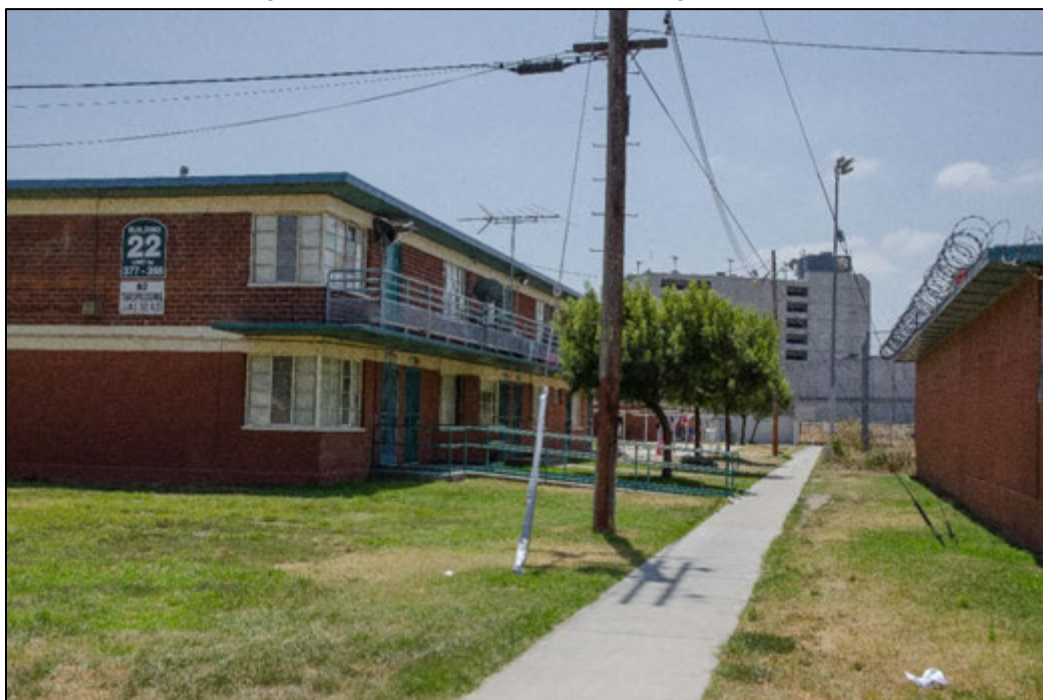
Figure 3.4-18. Key View #1b – Existing Conditions
