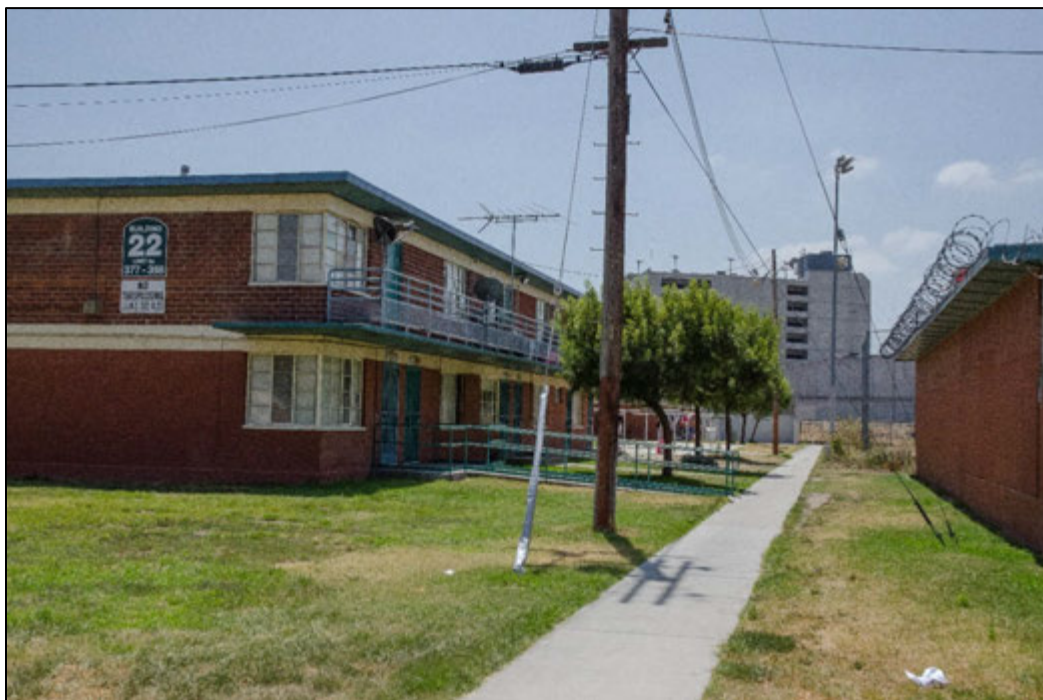
Figure 3.4-20. Key View #1b – Existing Conditions
