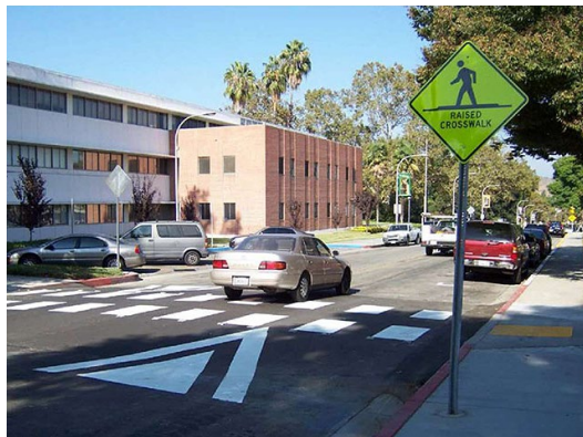
Raised pedestrian crossing
