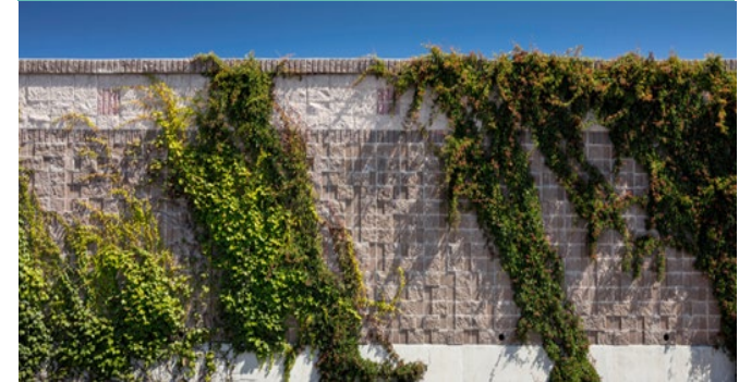
Sound Wall Improvements
