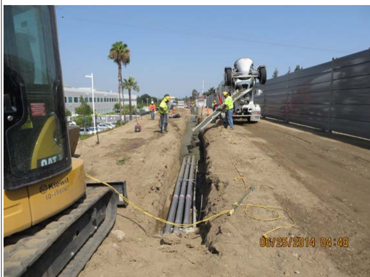
Segment 2: Ductbank work between Huntington and 5th
