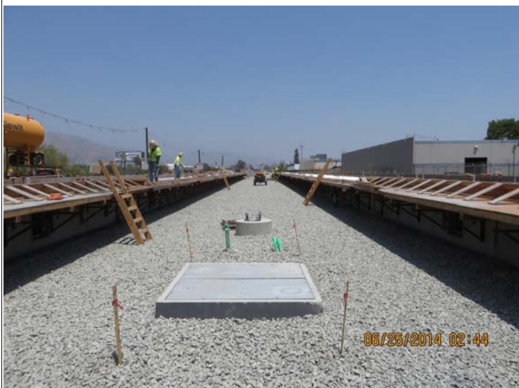
Segment 4: Irwindale Station - Deck Forming Work
