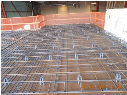
Steel rebar reinforcement at mezzanine level at Bldg. 1.
