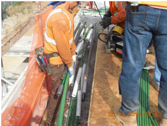
Repair of cables at deck roof level at Ramp #3.
