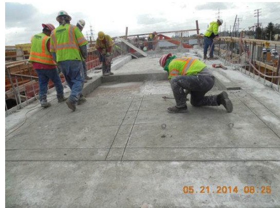
2 nd phase of surgical concrete demo at ramp deck.
