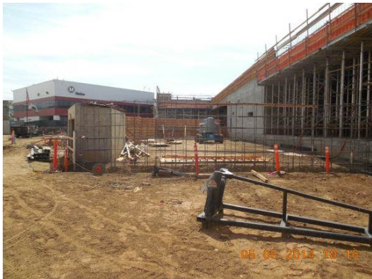
Rebar placement for cast-in-place walls at CNG Yard.
