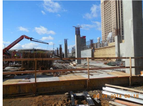
Formwork at shear walls at the Administration Building.
