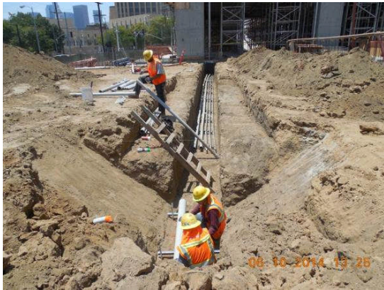
Placement of UG conduits to the DWP Utility Yard.
