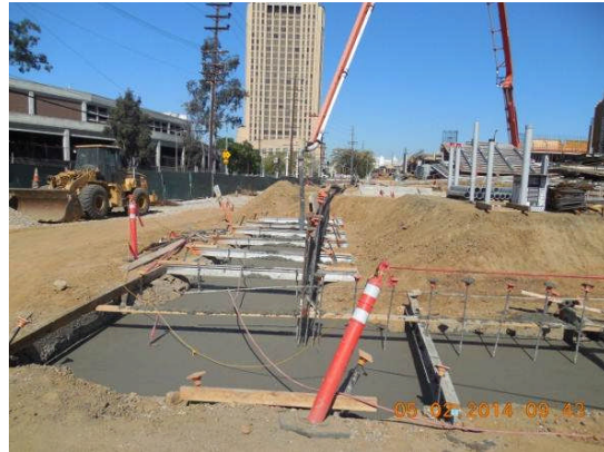
Concrete poured at footings of DWP Utility Yard.
