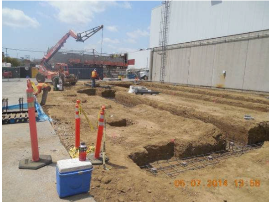
Rebar placement for foundation at chassis wash area.
