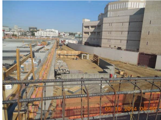
View of completed screen walls #1 and 2 at CNG Yard.
