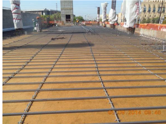
Rebar placement at Level 1 at Transportation Bldg.
