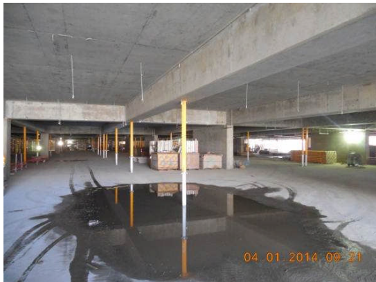
View of lower level Parking Garage.
