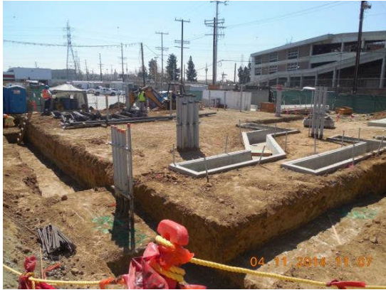
Excavation for footing at DWP Utility Yard.
