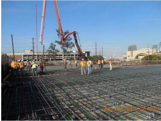
Concrete placement at Roof Deck No. 14, Building B.
