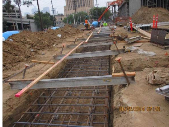
Placement of concrete at wall foundation for the Tire Shop.
