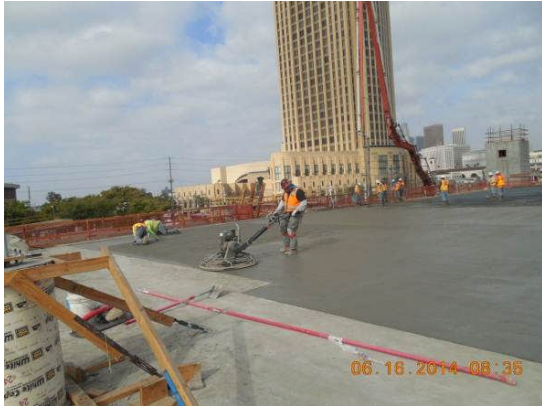
Concrete finishing of roof level Deck #18 at Parking Garage.
