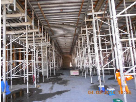
Shoring upper decks slabs/beams at Garage Bldg. Area.
