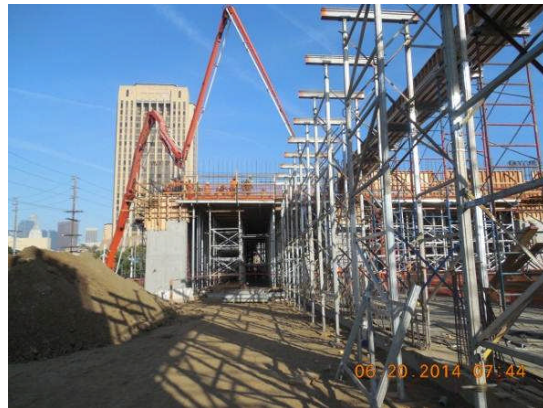
Concrete pouring of roof level Deck #14 Building B.
