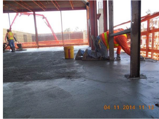
Finishing of concrete slab at mezzanine level in Bldg. 1.
