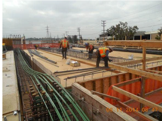
Reinstallation of steel and tendons in roof level Deck #14.
