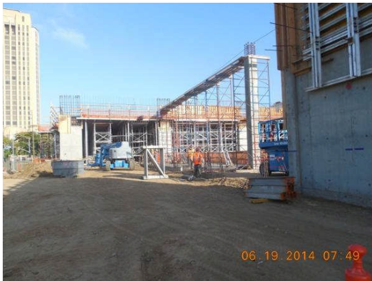
Side view of reconstructed roof level Deck #14 Building B.
