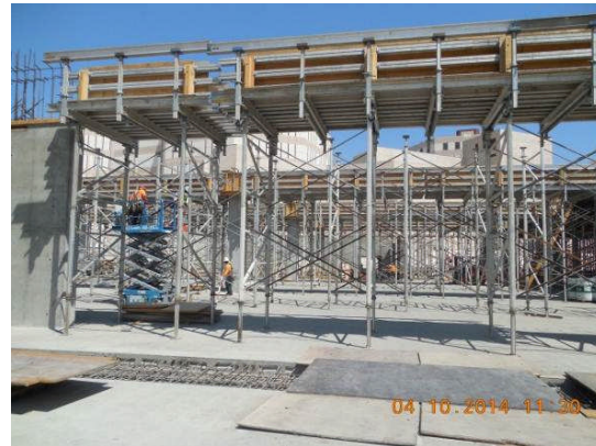
Shoring and beam formwork for upper level decks at Garage.
