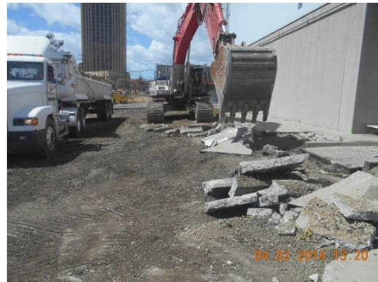
Chassis wash area existing AC slab demolition.
