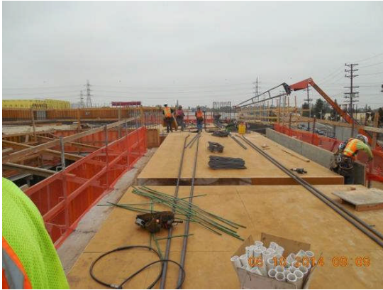
Panel deck reinstatement at roof level of Deck # 14.
