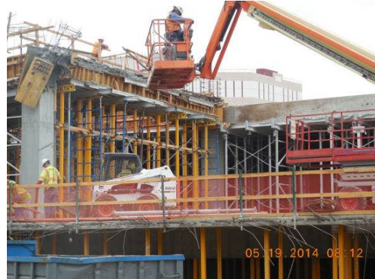
Concrete demo on ramp that was poured with Deck #14.
