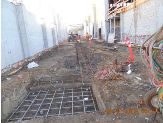
Steel rebar placement for footings at Areas 9 & 10.
