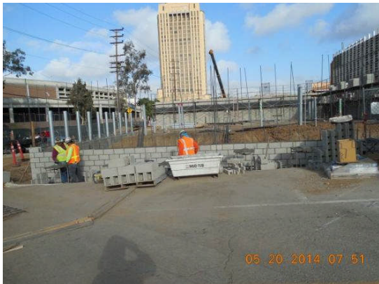
Placement of CMU walls at DWP Utility Yard.
