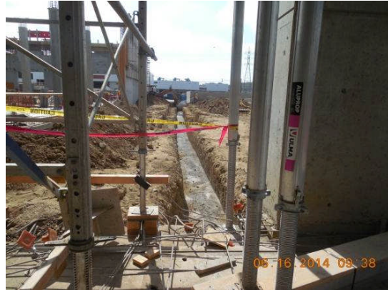
Concrete slurry to the UG elec. conduits to the DWP Yard.
