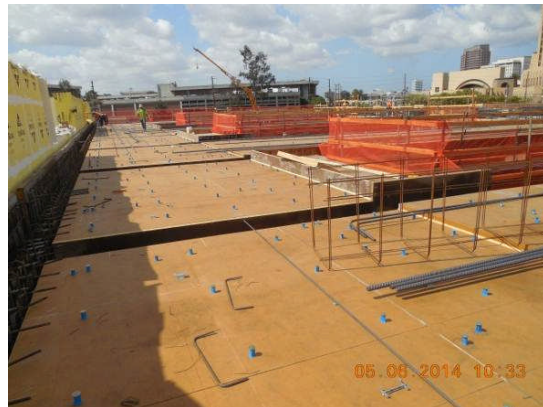
Roof Deck #1 rebar placement at Maintenance Building.
