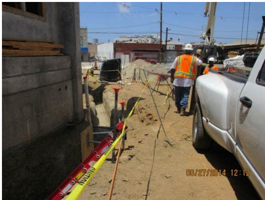
Placement of 6" gas line to the CNG Yard at Metro Drive.
