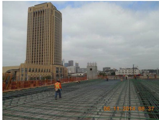
Placement of steel rebar at roof level decks Parking Garage.
