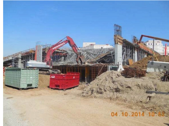
Surgical demolition of collapsed upper Deck #14.
