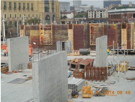
Placement of steel reinforcement at stern wall Level 1 Area 2.
