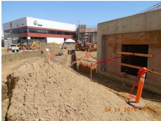
Excavation of footing at CNC Yard.
