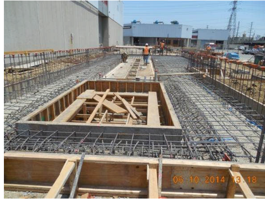
Steel reinforcement for footings at chassis wash area.
