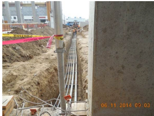
Placement of UG conduits for the DWP Utility Yard.
