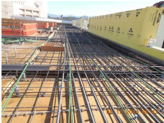
PT cables /rebar reinforcement of roof level at Bldg. 1.
