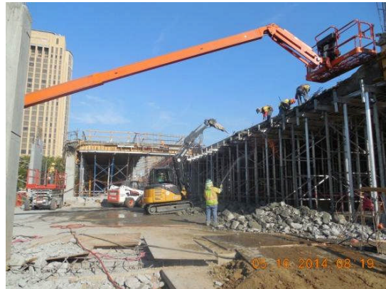
1 st phase surgical demo of collapsed upper Deck 14.
