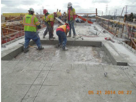
Concrete slab saw cutting and demo ramp Deck 2 nd phase.
