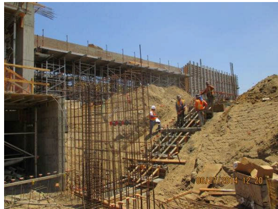
Installation of steel reinforcement at the East stairs Bldg. C.
