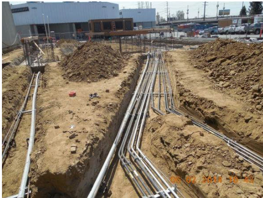
Placement of elec. UG conduits at chassis wash area.
