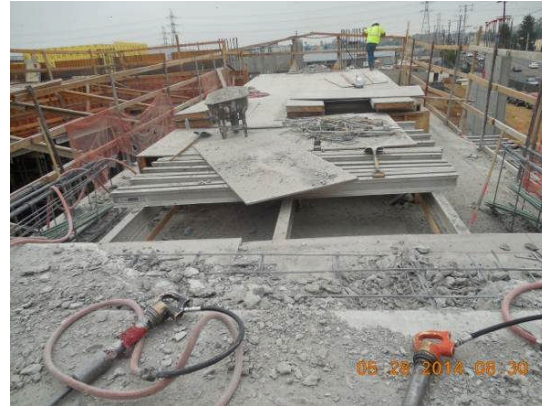
Concrete slab demolition at CJ ramp Deck 2 nd phase.
