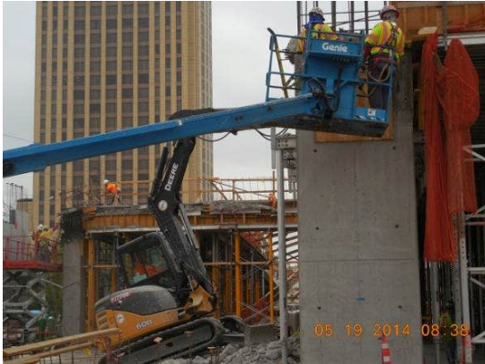
Surgical demolition of concrete around columns of Deck 14.
