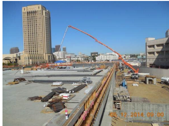
Concrete placement at upper level Deck# 17 at Parking Garage.
