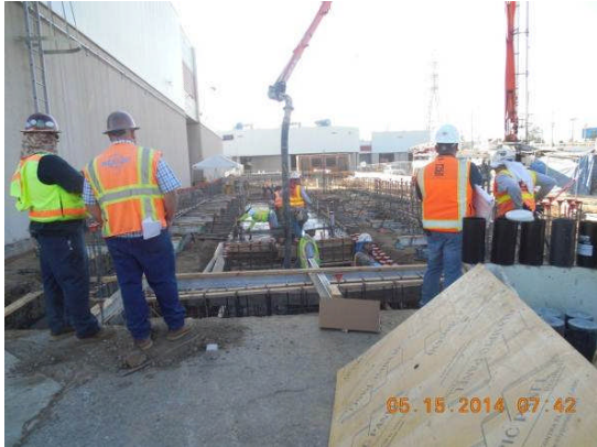
Concrete placement for foundation at chassis wash area.
