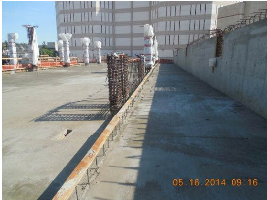
View of finished level 1 at Transportation Building.
