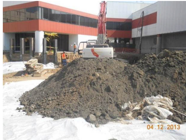
Removal of SC Gas Company hazardous soils.
