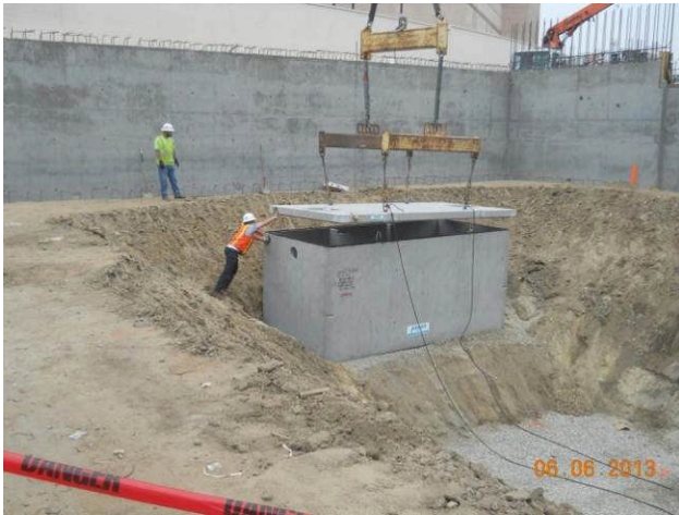
Underground oil interceptor installation
