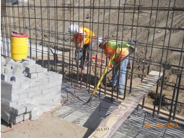
Reinforcement at walls of Parking Garage.
