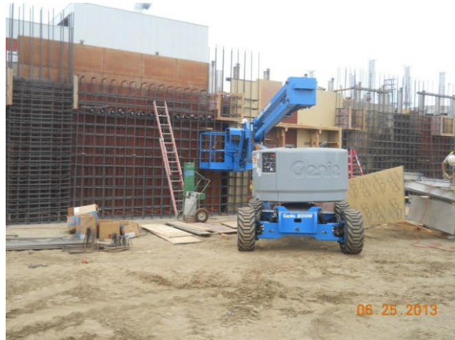
Concrete wall formwork and reinforcement.
