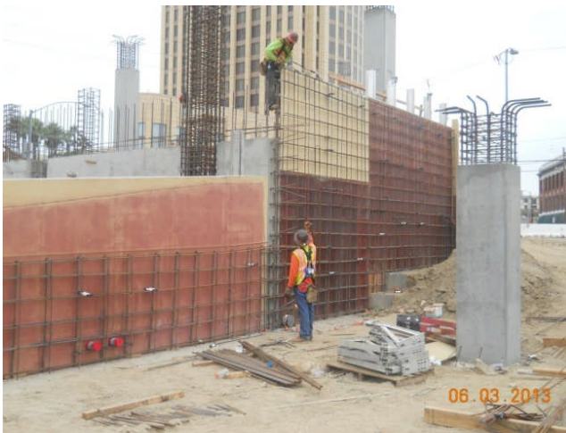
Wall formwork and reinforcement.
