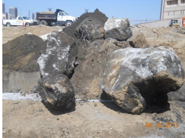
Removal of existing concrete obstructions.
