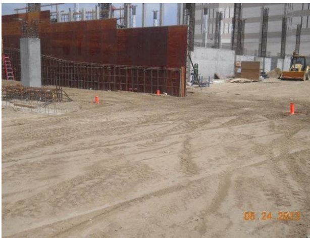
Wall formwork at lower level Parking Garage.
