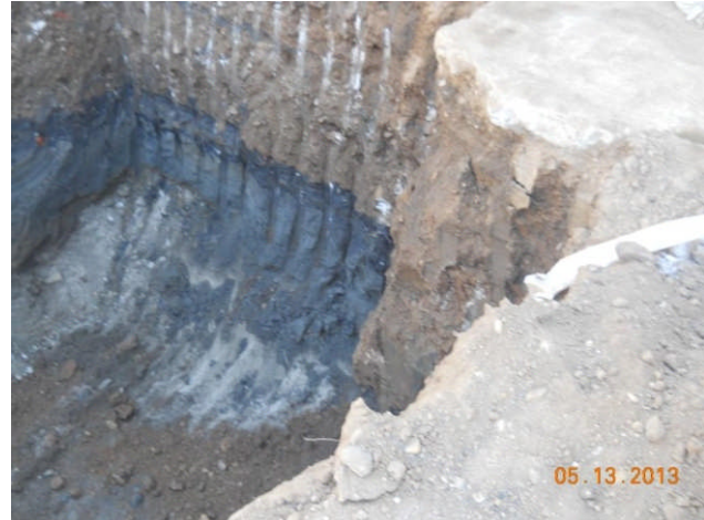
Removal of SC gas hazardous soils.
