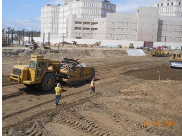
Earthwork at east side of Lyon Street.
