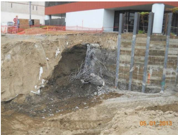
Excavation at adjacent to Diamond Building.
