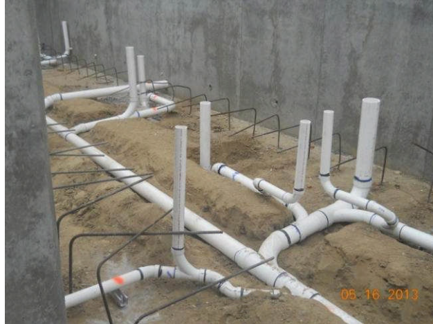
Under slab plumbing rough-in work.
