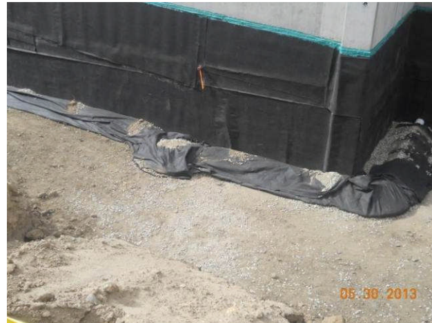
Water proofing and drainage at walls.
