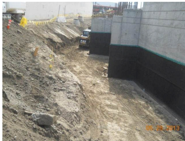
Water proofing of exterior walls.
