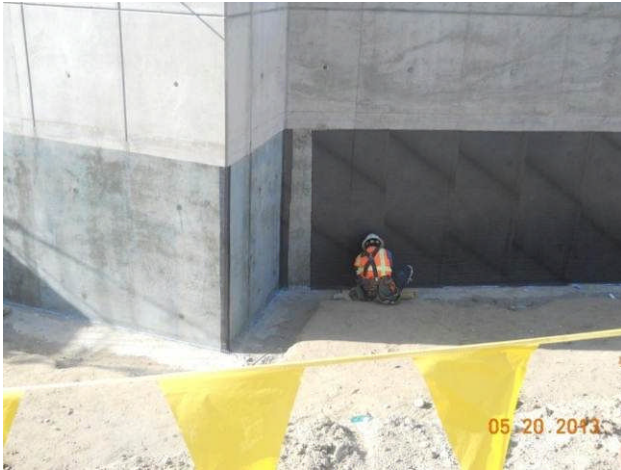
Water proofing of exterior walls.
