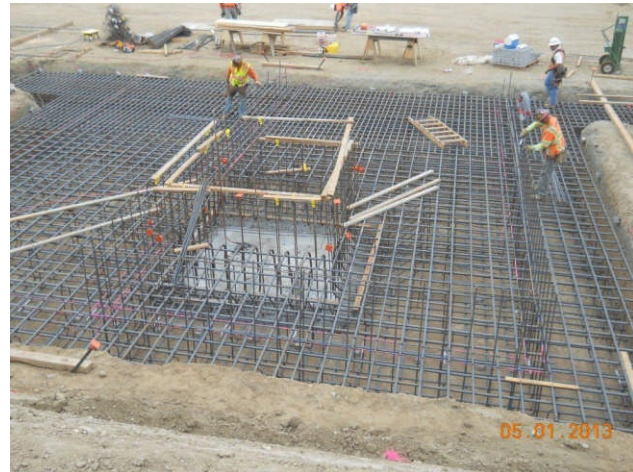
Foundation reinforcement at Parking Garage.
