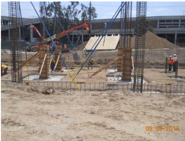
Column formwork at Parking Garage Building.
