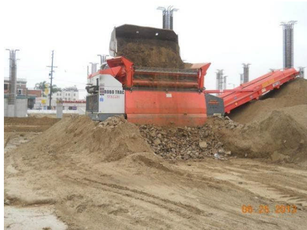
Screening of imported soil for rocks and debris.
