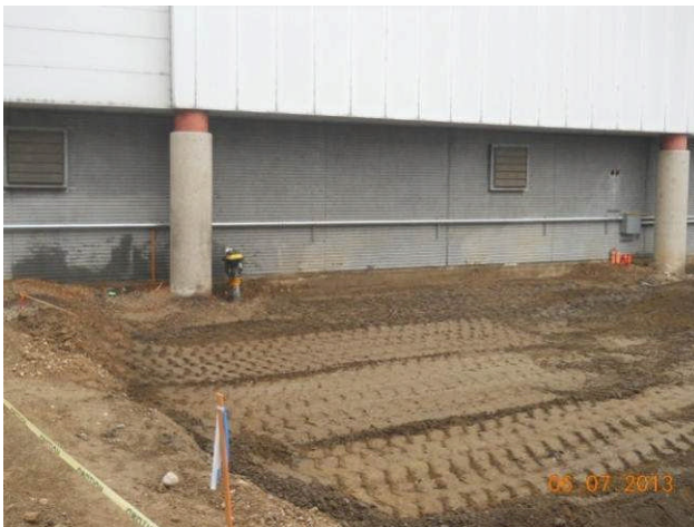
Compaction of earthwork at Building 1.
