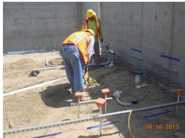
Concrete formwork at Administration Building.
