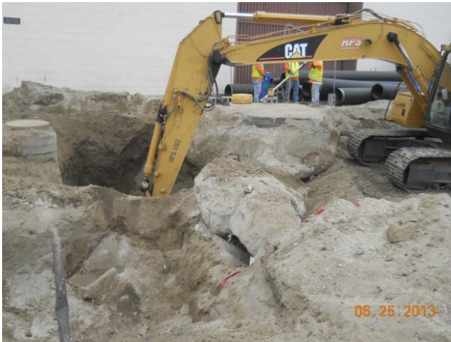
Connection of underground storm drain line.
