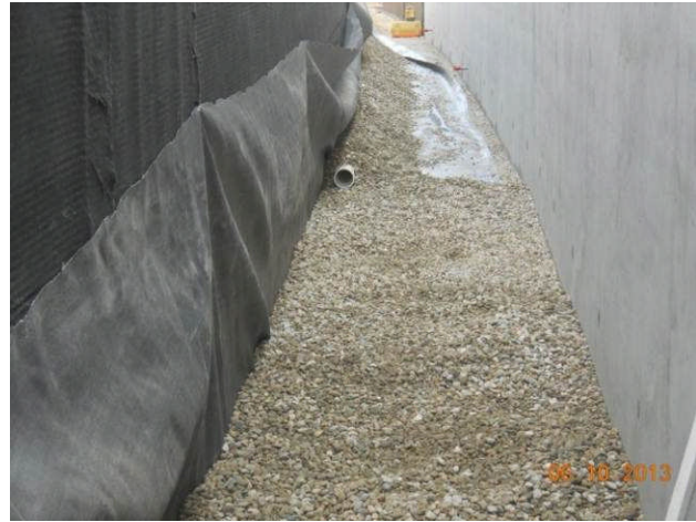
Drainage system at building walls.
