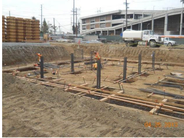
Foundations and columns at Maintenance Bldg.
