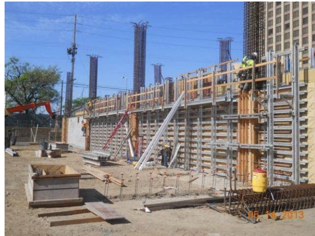
Lower level wall formwork at Parking Garage.
