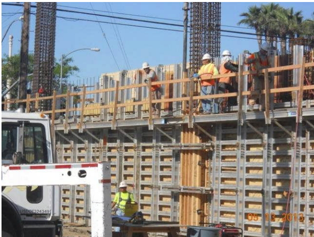
Concrete placement at Parking Garage walls.
