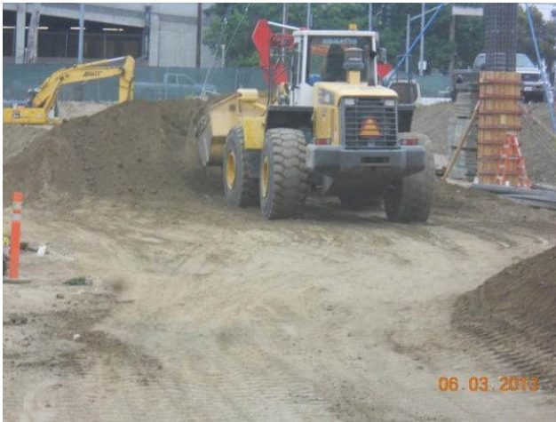
Import of structural fill.
