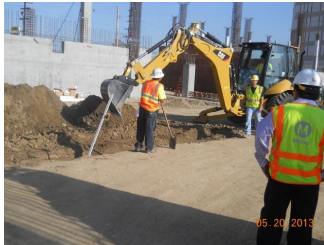
Fiber optic trenching at Vignes Street.
