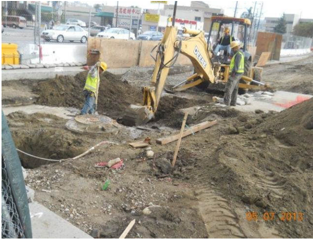
Fiber optic system on Vignes Street.
