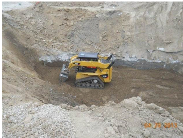
Excavation adjacent to Diamond Bldg.
