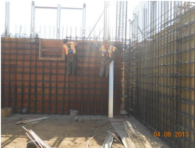
Concrete reinforcement installation.
