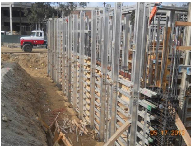
Wall formwork at lower level Parking Garage.
