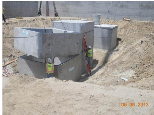
Underground oil interceptor installation.
