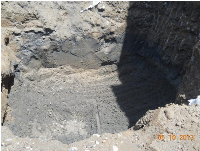
Removal of SC gas hazardous soils.
