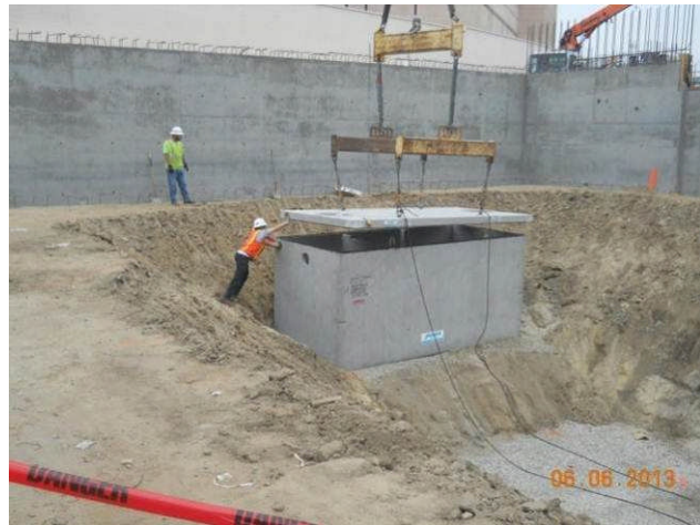
Underground oil interceptor installation.
