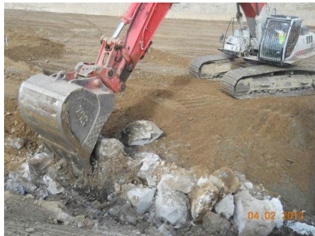
Removal of concrete obstructions.
