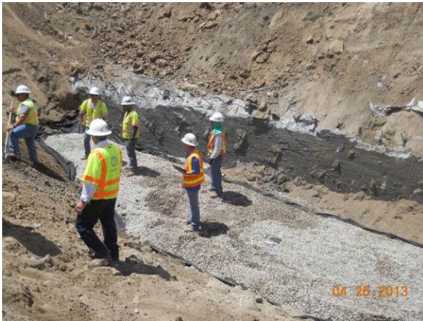
Excavation adjacent to Diamond Bldg.
