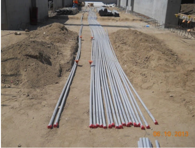
Underground electrical rough-in.
