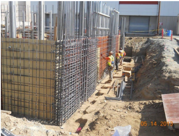
Wall reinforcement at Maintenance Building.
