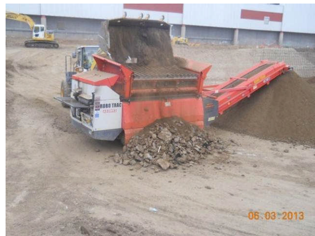
Screening of soils for rocks and debris.
