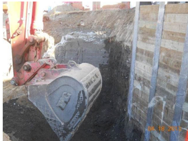
Excavation adjacent to Diamond Bldg.
