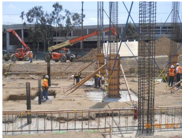
Column formwork at parking Garage Building.
