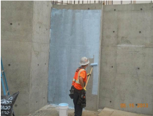
Waterproofing of exterior walls.
