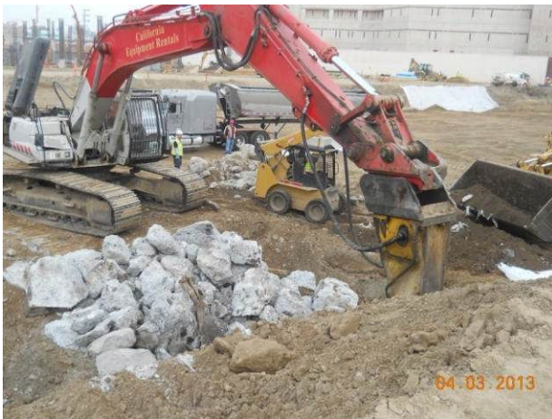
Removal of underground concrete obstructions.
