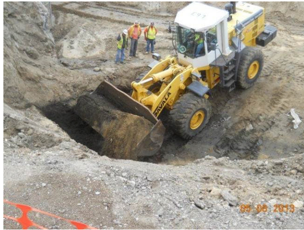
Removal of SC Gas hazardous soils.
