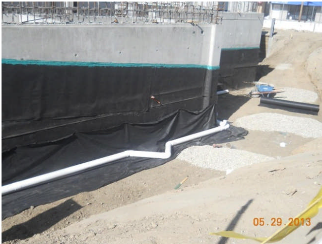
Water proofing and drainage at walls.
