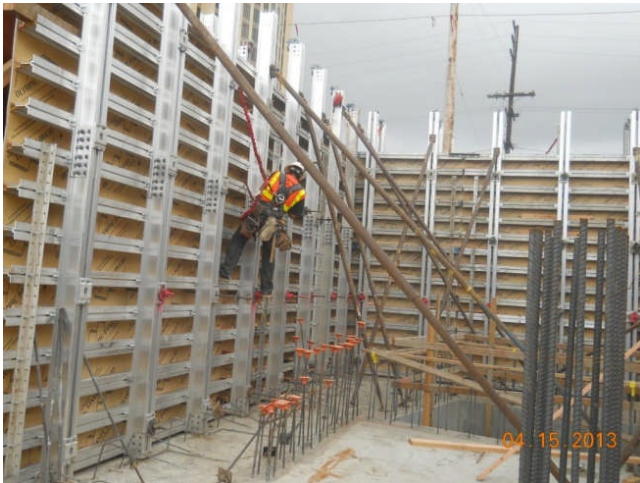
Foundation reinforcement at Admin. Building.
