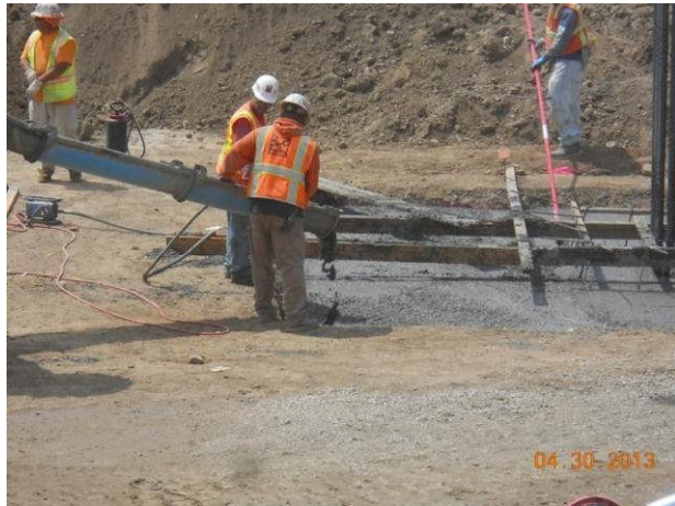
Foundation excavation at Parking Garage.
