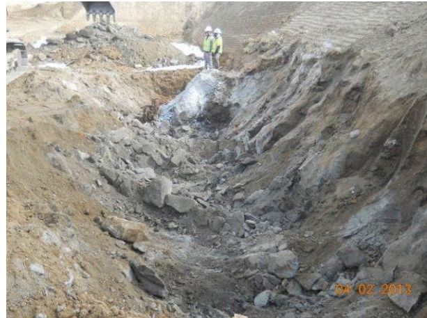
Removal of underground concrete obstructions.
