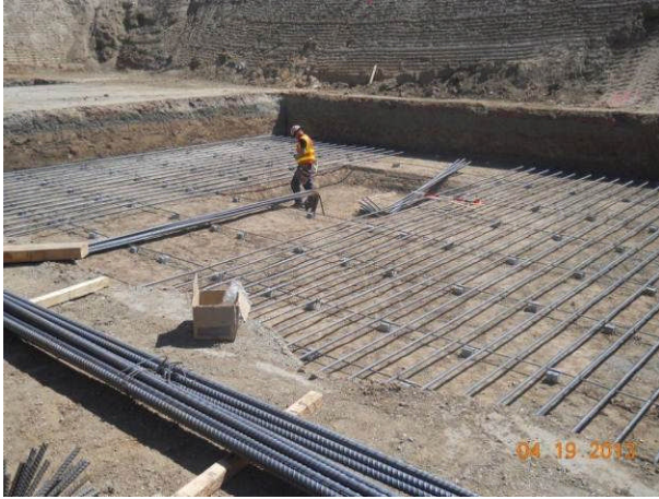
Reinforcement at Maintenance Bldg.
