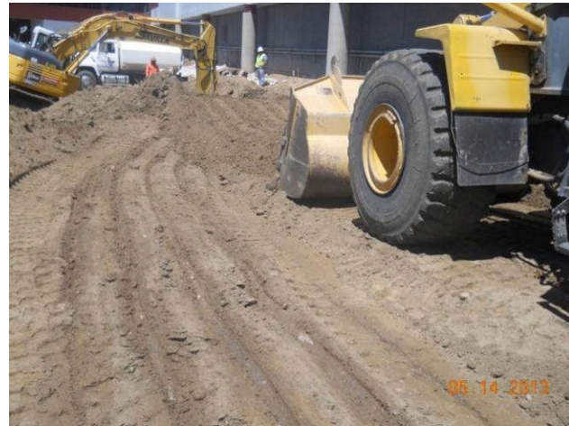
Slot cutting adjacent to existing Building 1.
