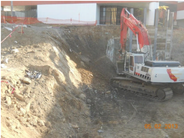
Excavation adjacent to Diamond Bldg.
