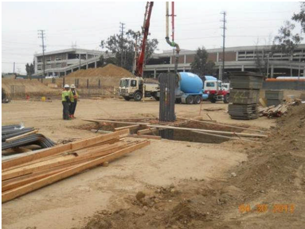
Foundation reinforcement at Parking Garage.
