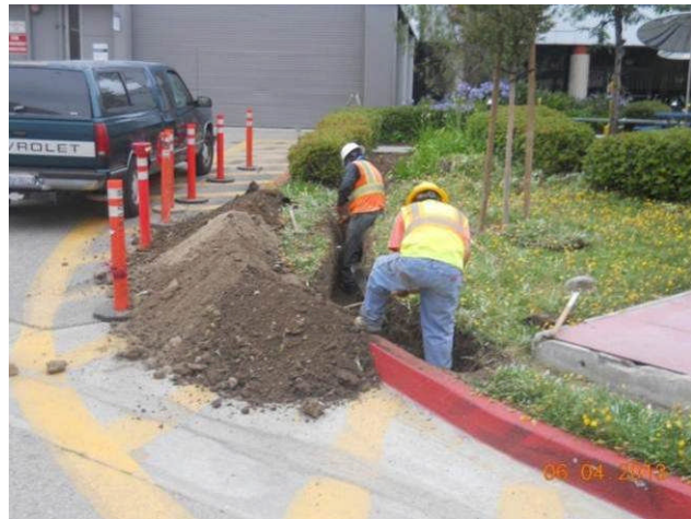
Connection of landscape irrigation line.
