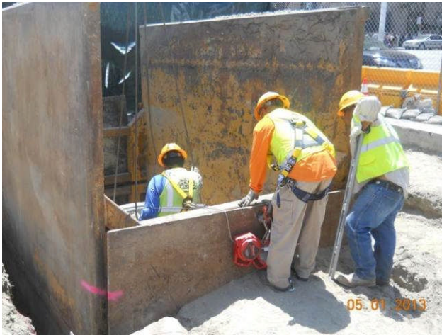
Vault installation for fiber optic system.
