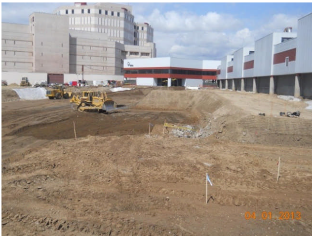
Earthwork at east side of Lyon Street.
