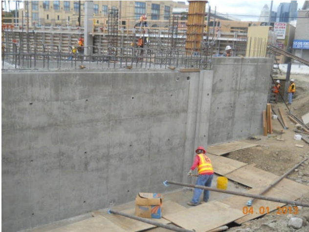
Formwork removal at Transportation Bldg.
