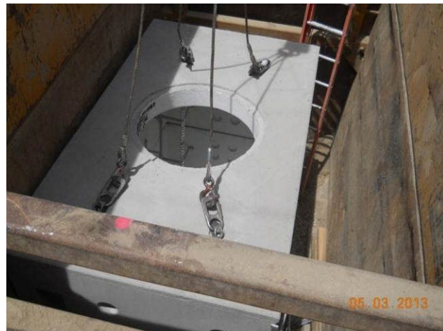
Fiber optic vault installation at Vignes Street.
