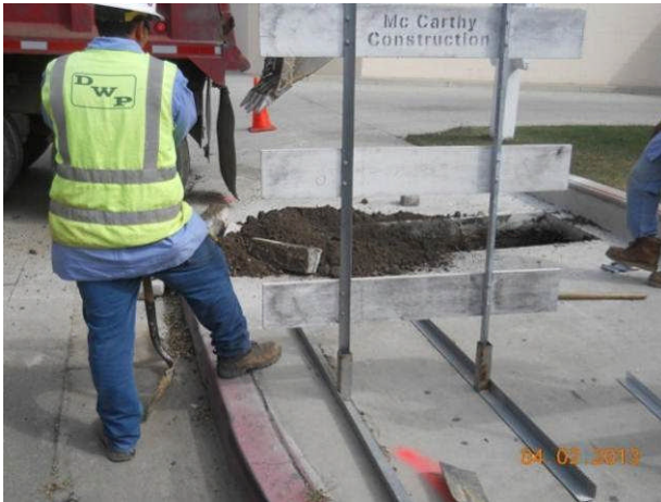
Excavation for water meters by LADWP.
