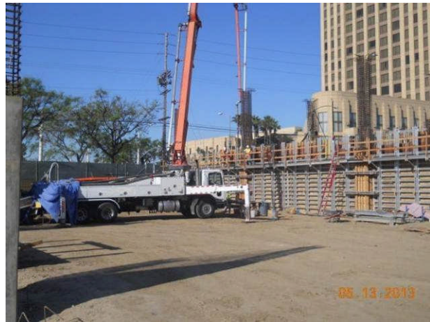
Concrete placement at Parking Garage walls.
