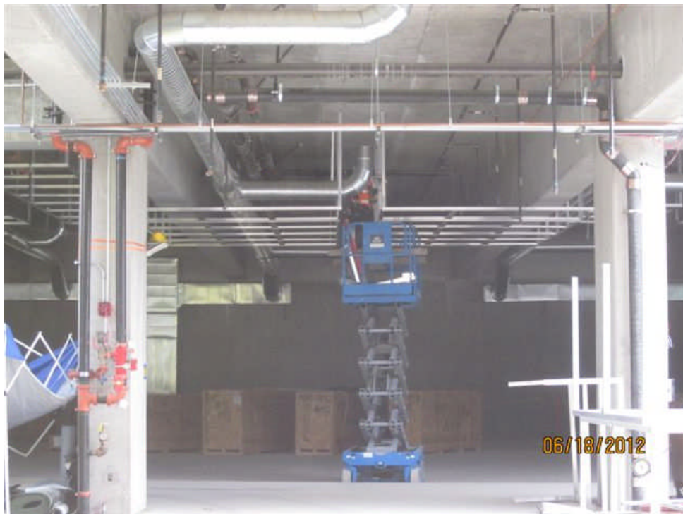
Installing metal ceiling frames on concourse level.
