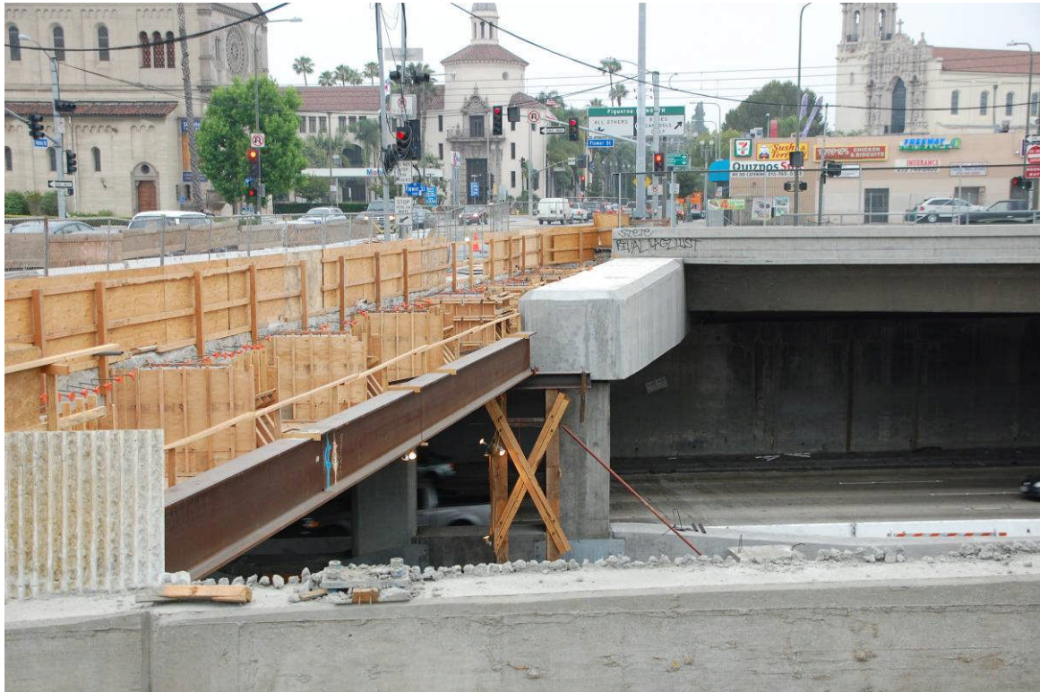
FW over NB traffic facing.
