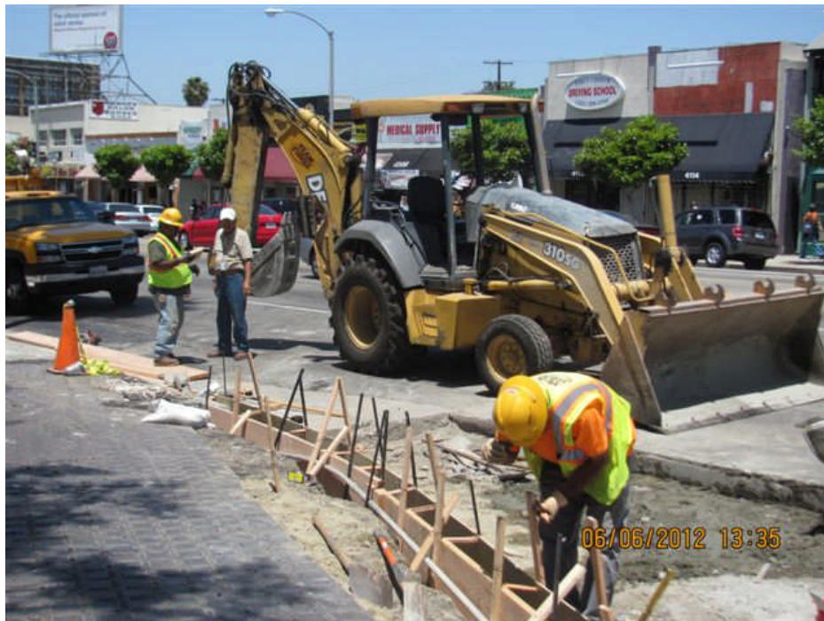
Restoration work at Crenshaw Blvd. and MLK Blvd.
