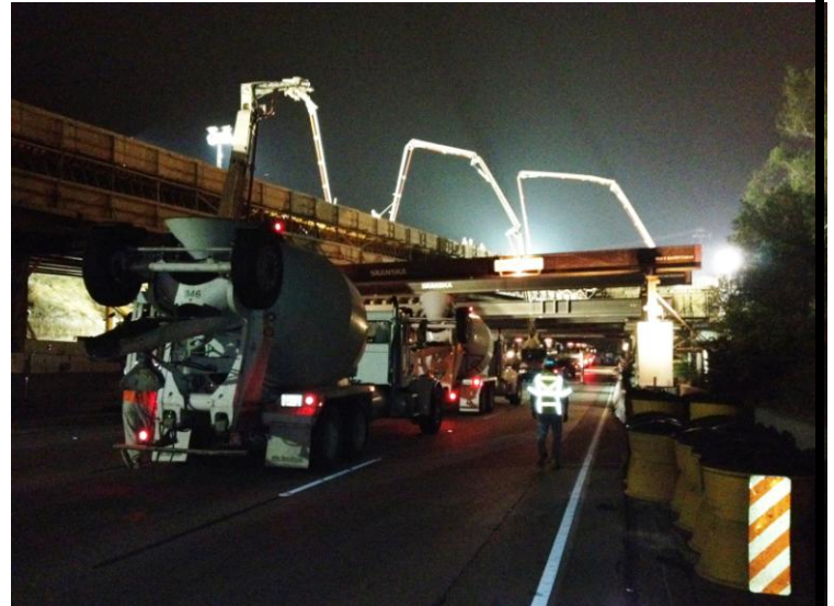
Nighttime Freeway Closure and Concrete Pour
