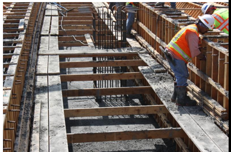
View of Bridge after Concrete Placement
