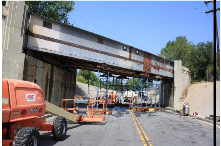
Prepping for Colorado Bridge demolition
