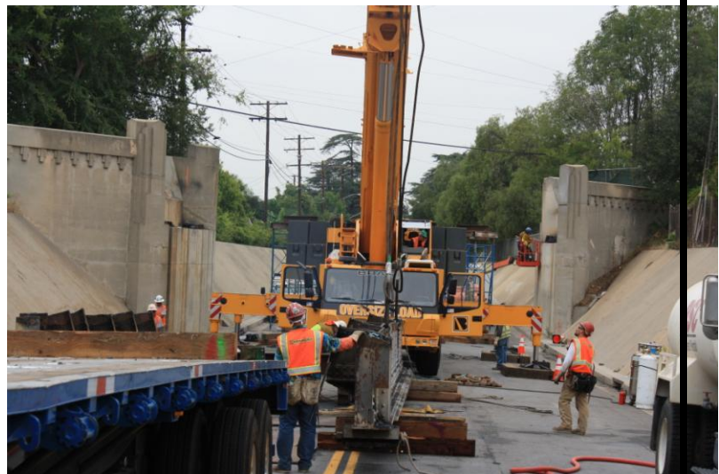
Post-demolition view of Colorado Bridge
