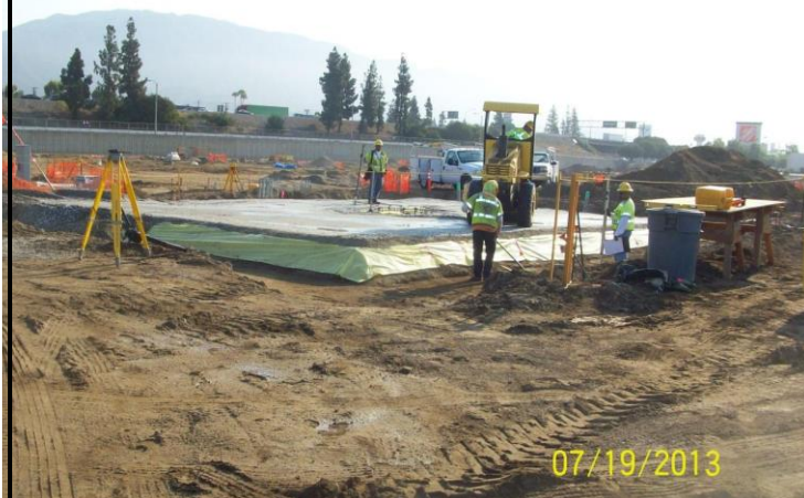
MOW building pad foundation base preparation
