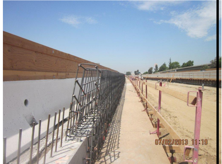
Barrier Wall Construction in Segment 1
