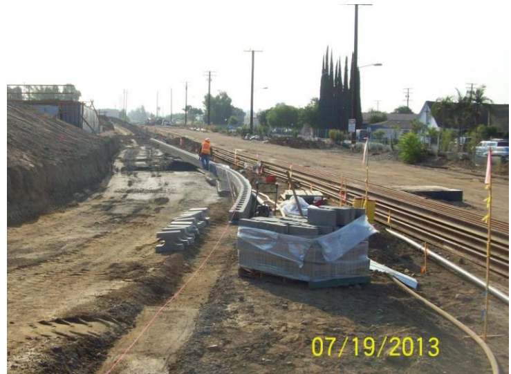
South Campus MSE Wall C
