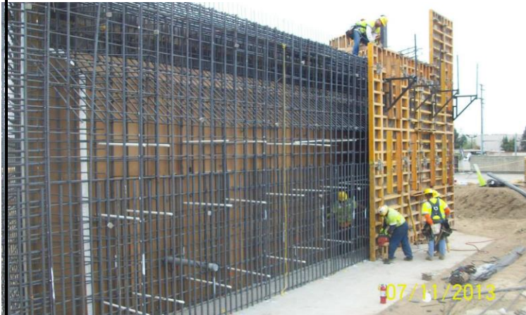
Santa Anita Bridge Abutment #3 Wall
