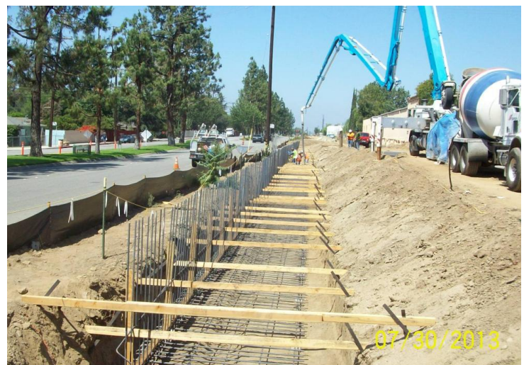
Duarte Road CMU retaining wall footing
