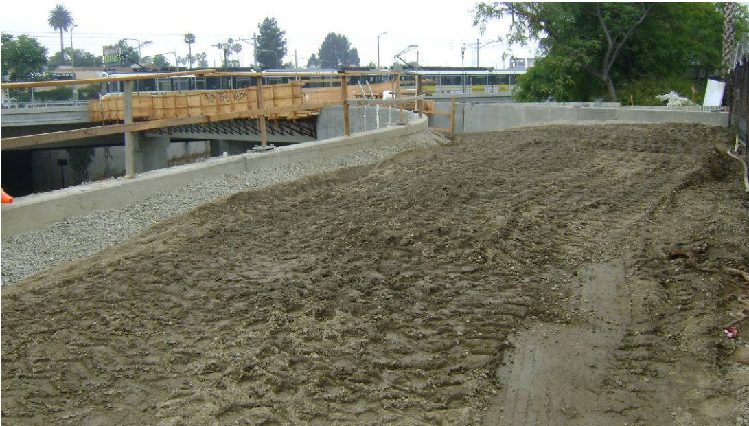
Plaza almost complete.
