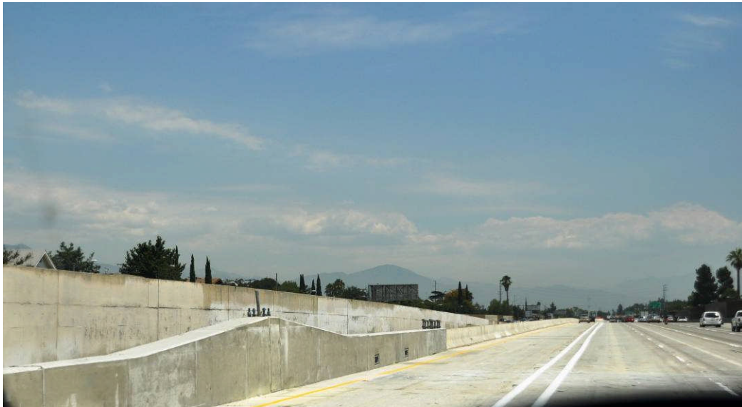
Median work at east end of I-10 Freeway.
