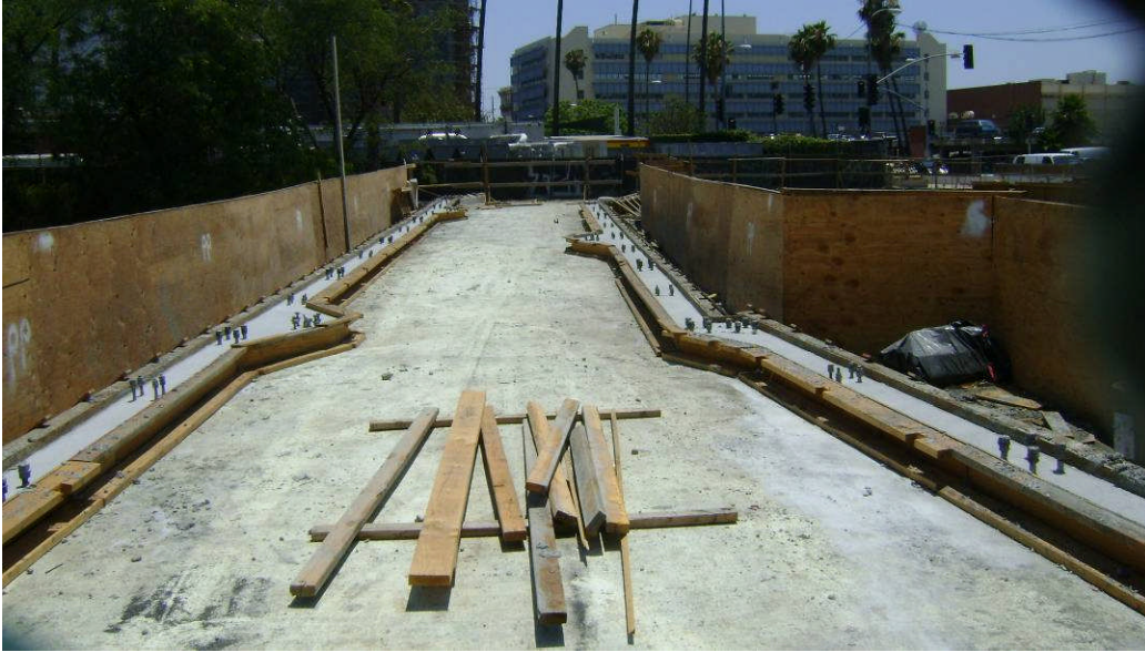
POC deck and curbs facing east.
