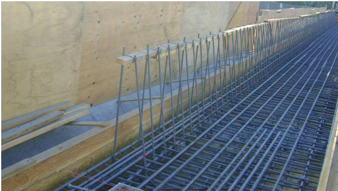
Facing east at Adams widening.
