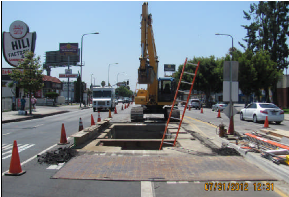
The Gas Co. relocating gas main at Exposition and Rodeo Ave.
