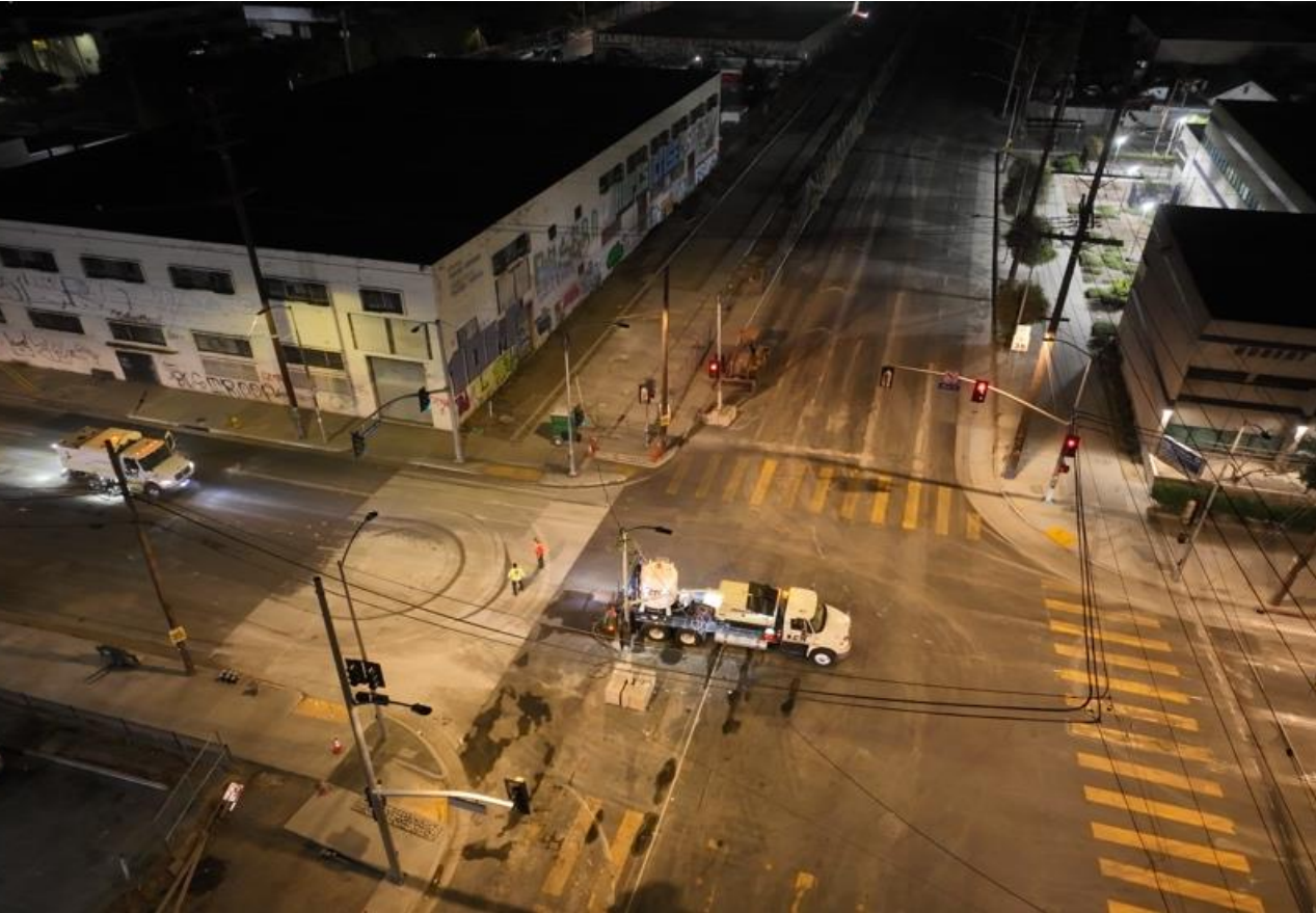
Main St Intersection Improvement Work completed
