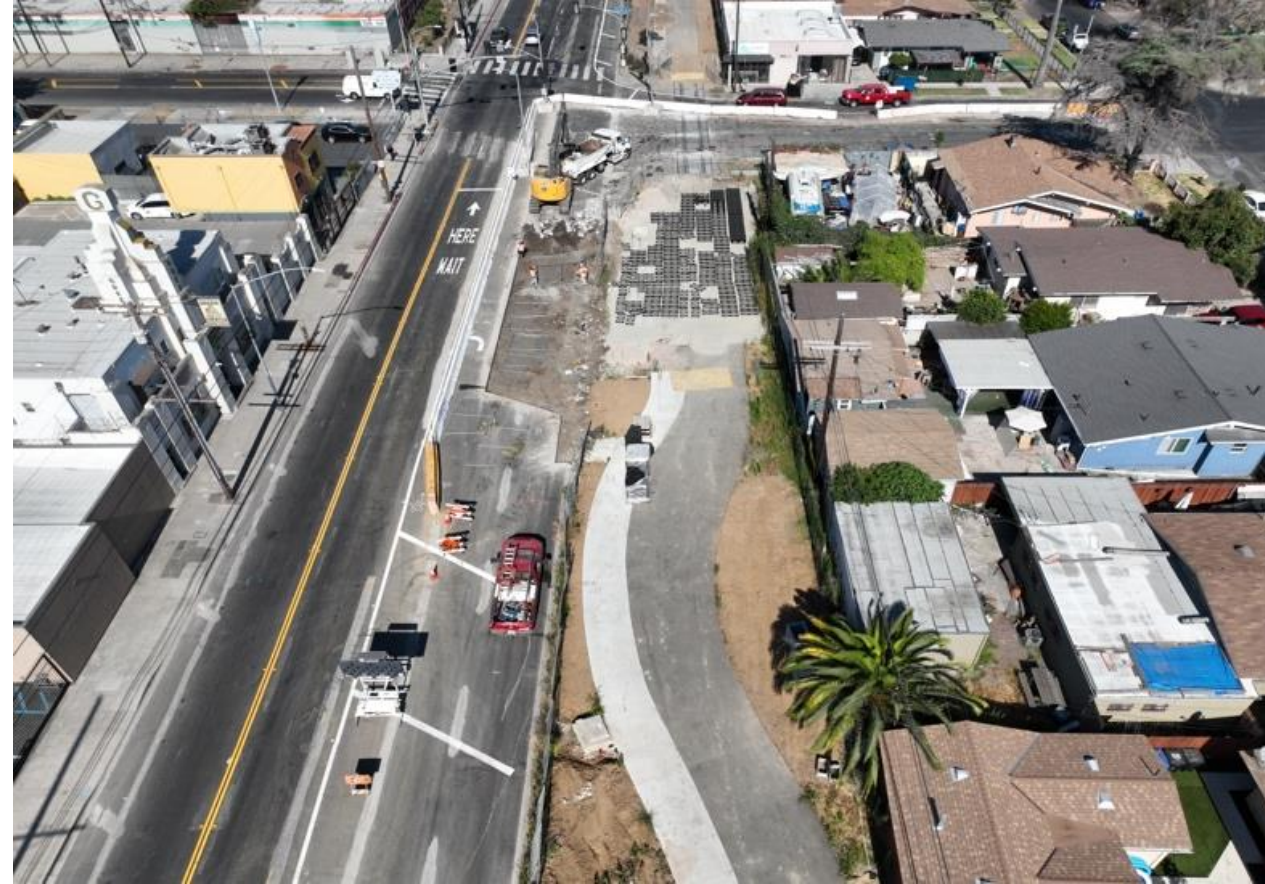
Removal of asphalt roadway, concrete bus-pad, and curb/gutter
