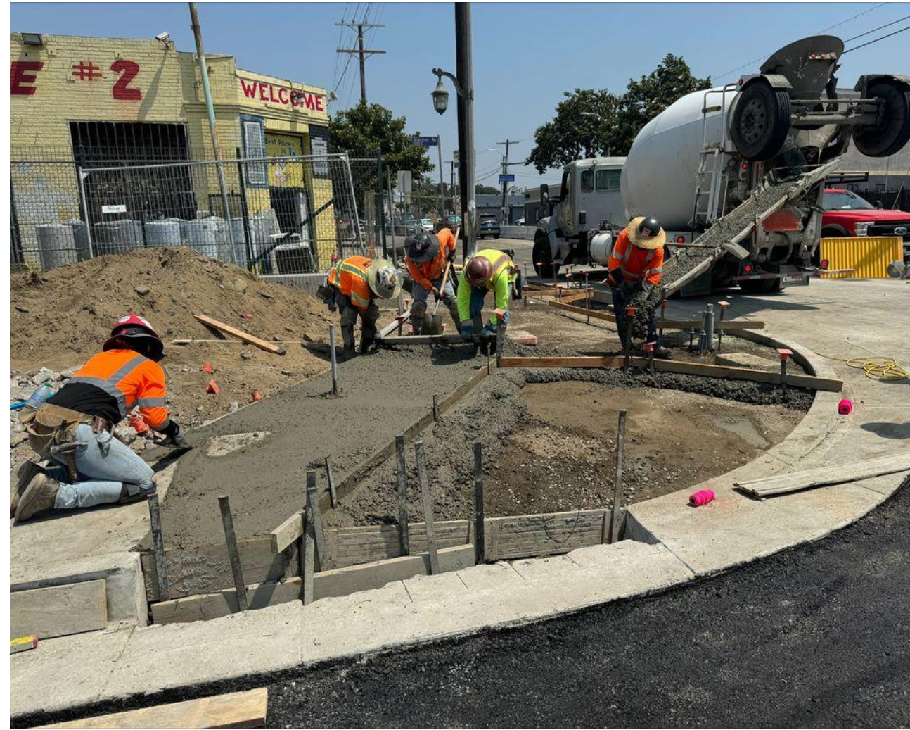
Paving, Sidewalk, Ramp
