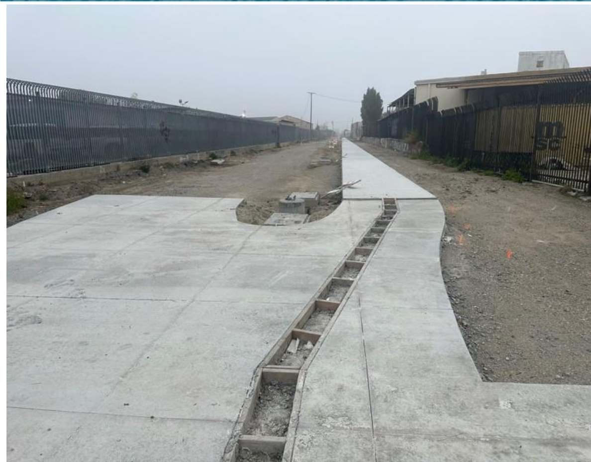
Mixing Zone Diagonal Segment: Bike and Pedestrian Path
