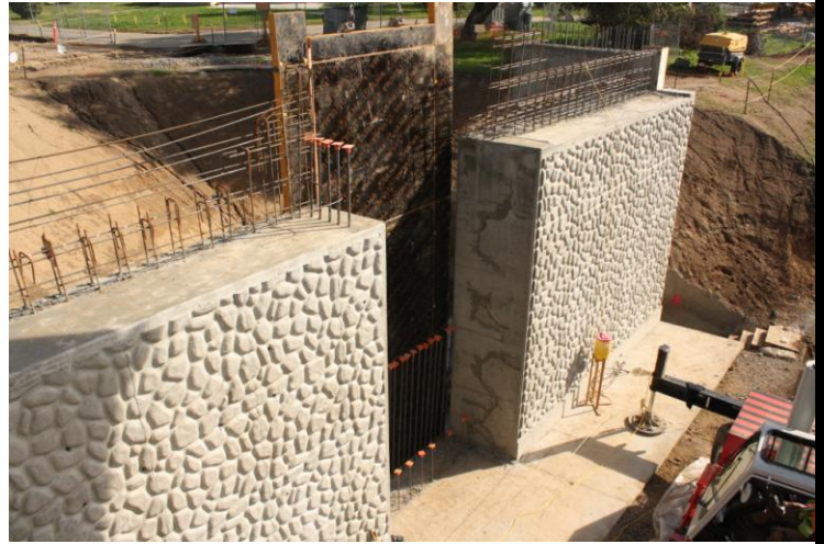
Work at Citrus Bridge
