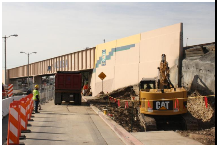
Work at Foothill Bridge
