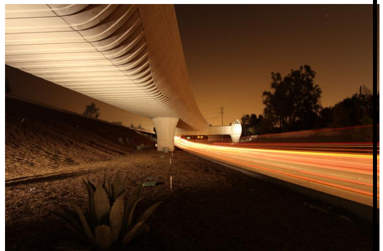
Nighttime view – soffit
