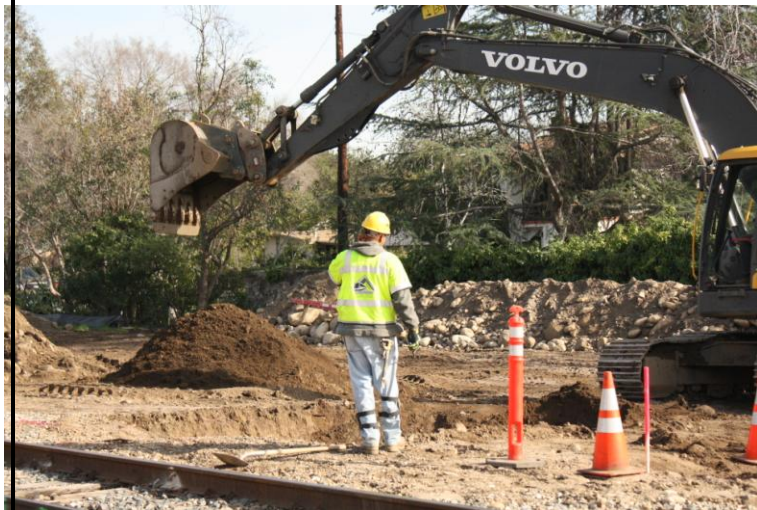
Grading in Segment 4
