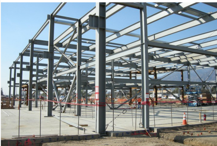
M&O: Main Shop Building Structural Steel
