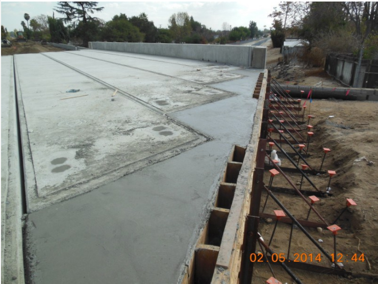
Segment 3: Santa Anita Wash Abutment 1 Backwall
