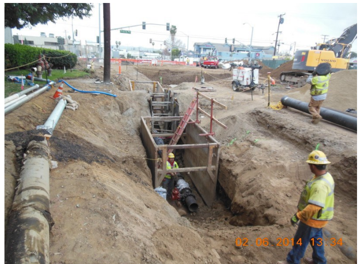
Segment 3: Waterline Work at Myrtle Avenue
