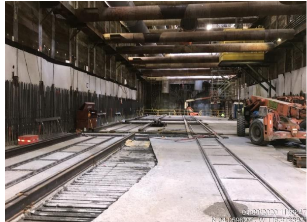
TBM Launch Box in Century City
