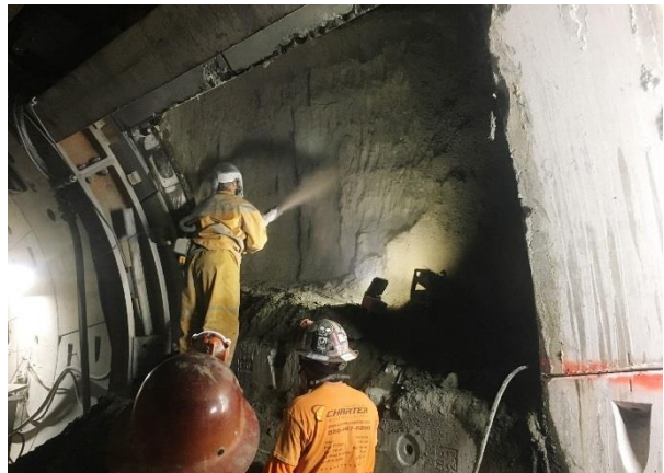
Reach 1 Cross Passage #11 Excavation
