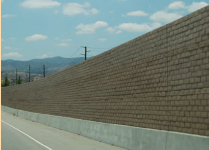
Existing Slump Stone Sound Wall along the Hasley Canyon SB on-ramp
