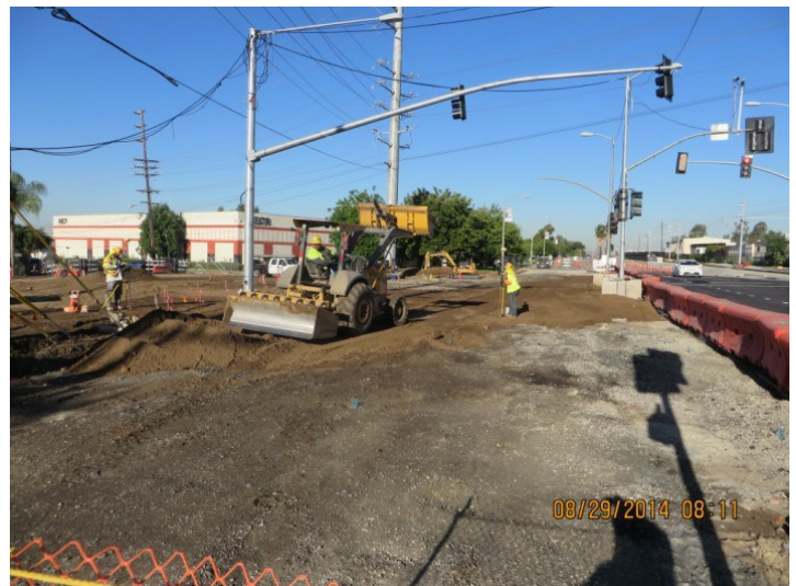
Segment 3: Mountain Ave - Rough Grading
