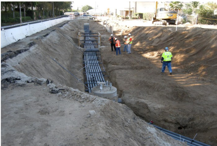
Operations Campus: Main Yard Track Lead - Ductbank Installation
