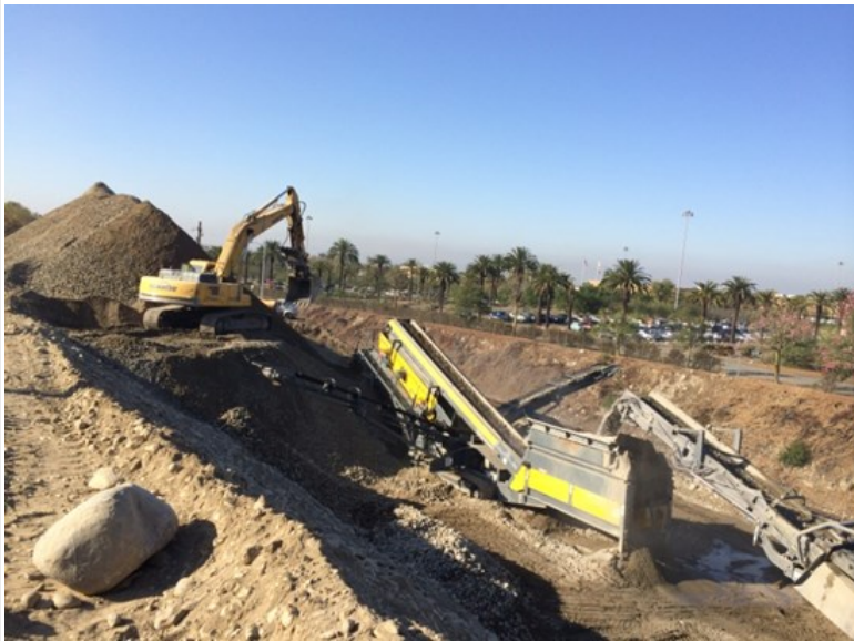
Irwindale Parking Structure Site Excavation
