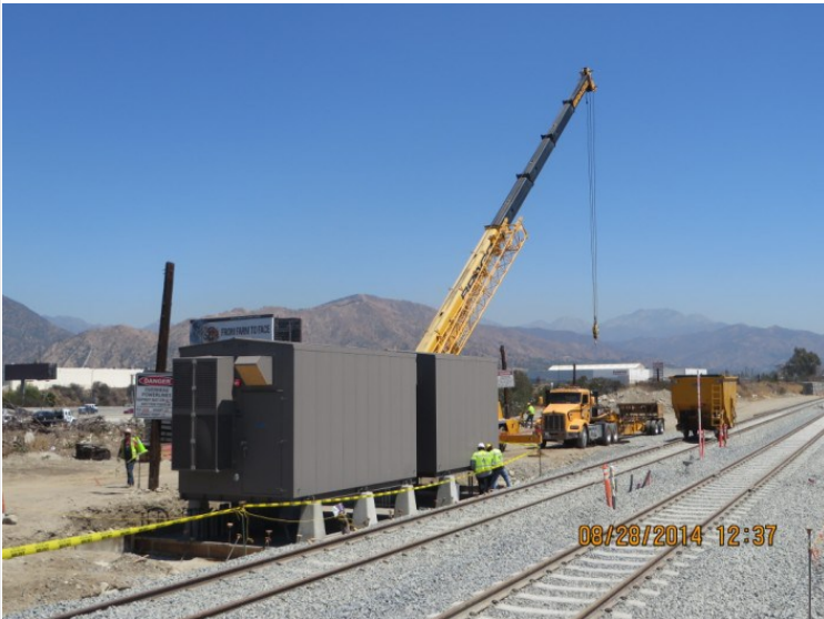
Segment 4: Irwindale Communications Bungalow Installation
