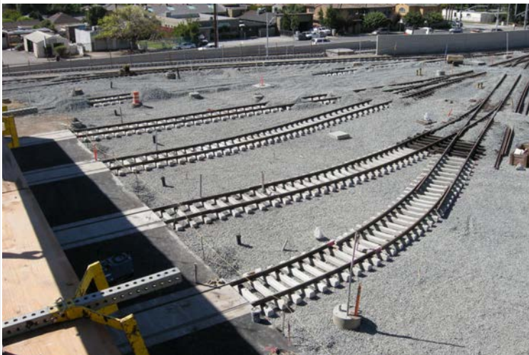
Operations Campus: Shop Lead Track Installations
