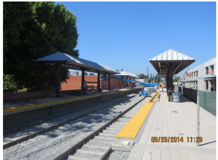
Segment 3: Monrovia Station - Canopy Roof Panel Installation
