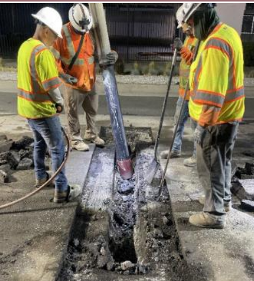
Trenching work activities
