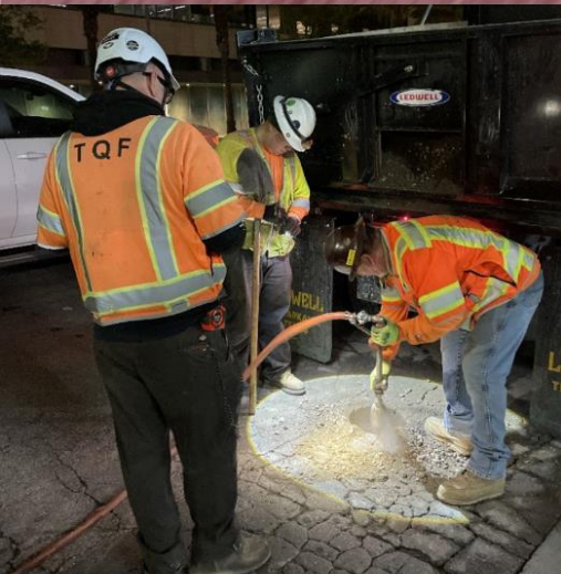
Potholing work activities
