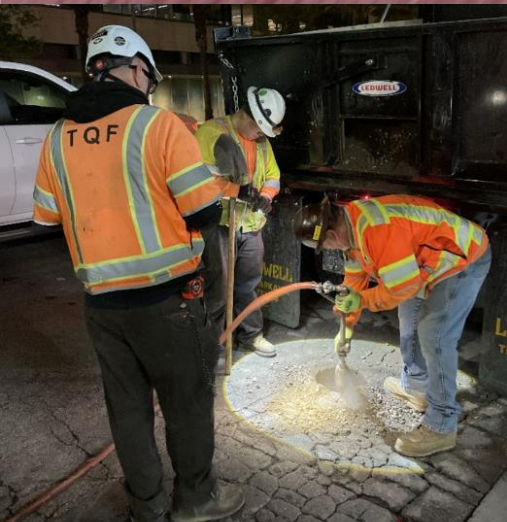
Potholing work activities
