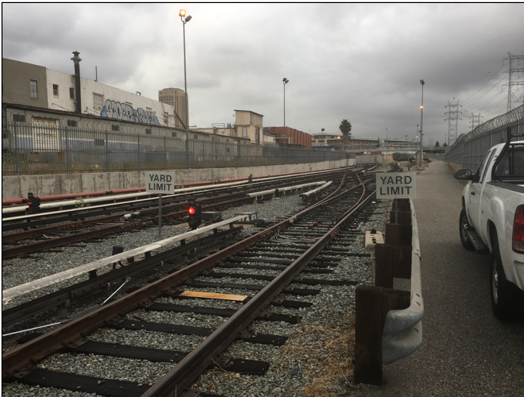
Figure 7. Segment of P-19-186804/P-30-176663 Within the Project Area, North of 1st Street Bridge; View Towards North.
