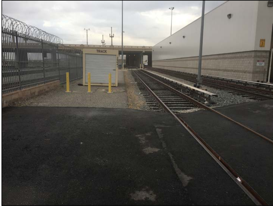
Figure 4. View of Northern Half of Project Area North of 1 st Street Bridge; View Towards South.
