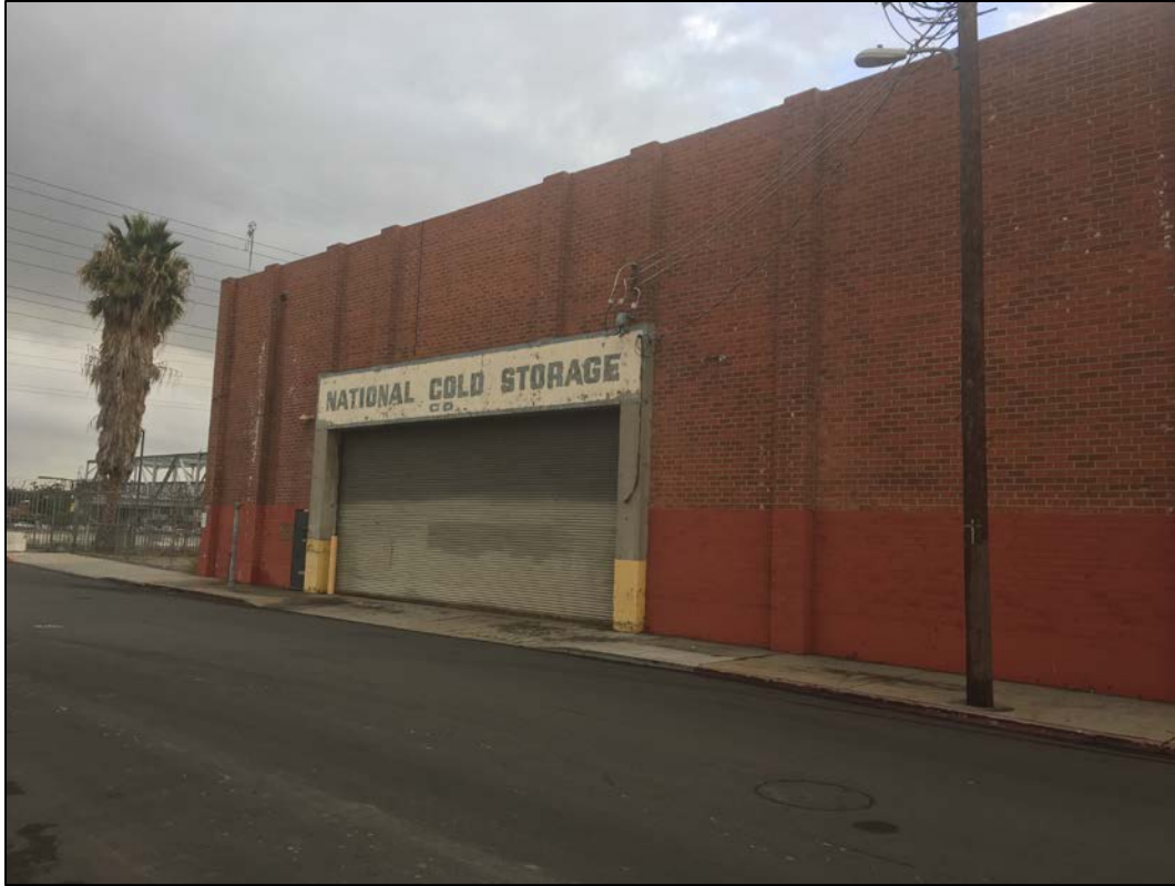
Figure 6. View of Cold Storage Building from Jackson Street; View Towards Southeast.
