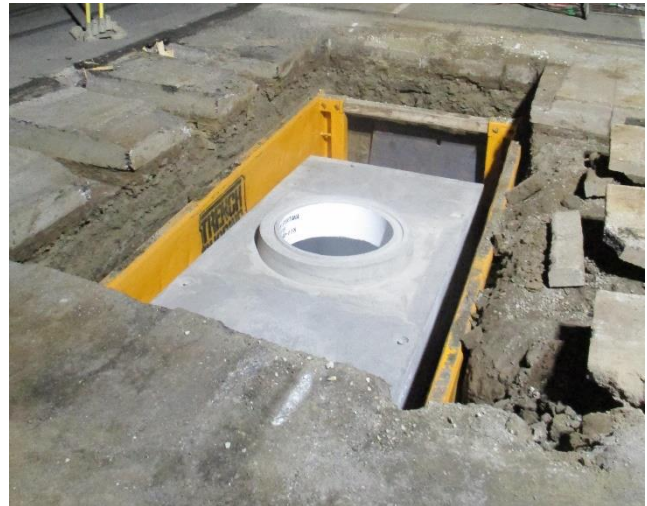
MH 800 on Wilshire Blvd. East of Federal
