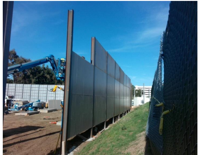
Soundwall Installation at VA Site
