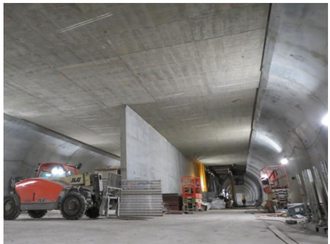
SEM Cavern post plenum placement
