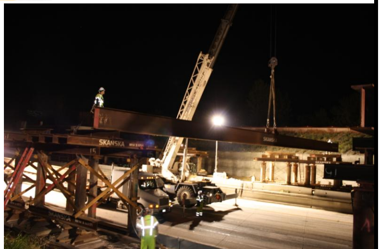
Nighttime freeway closure for Falsework erection
