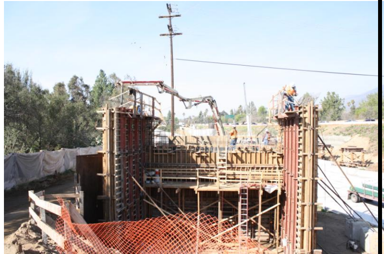
Concrete pour at South Abutment
