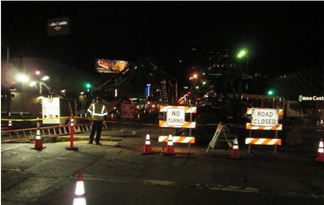
Nighttime Work at Wilshire/La Brea Intersection by the C1048 AUR Contractor
