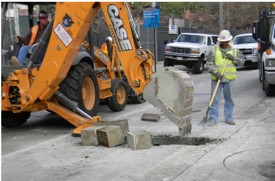
2 nd Street and Broadway – Gas Company Utility Work
