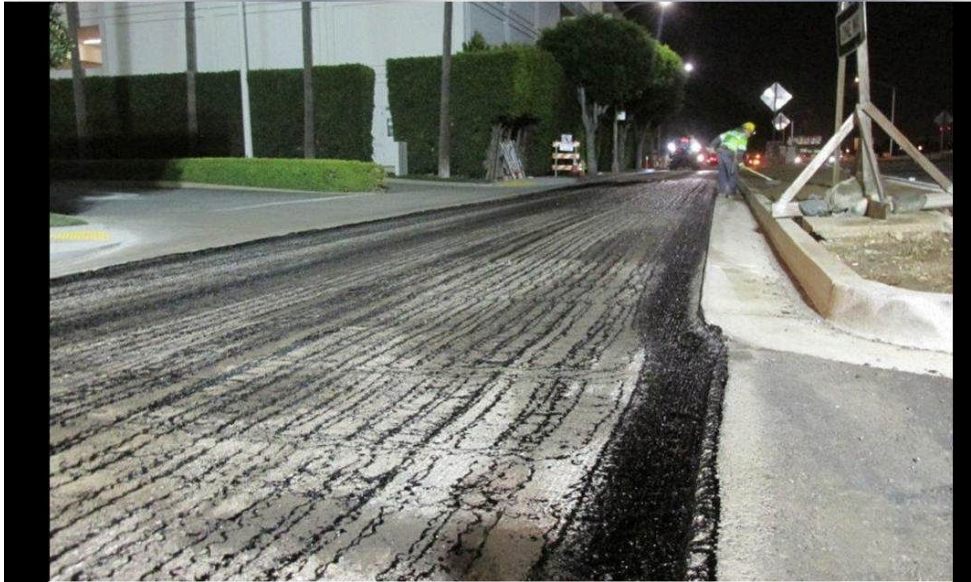
TACK COAT PRIOR TO ASPHALT CAP AT SANTA MONICA OFF RAMP AND COTNER AVE
