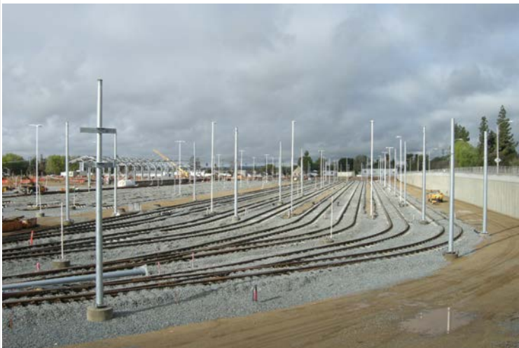
Operations Campus: OCS and Site Lighting Poles erected throughout the North Storage Track areas
