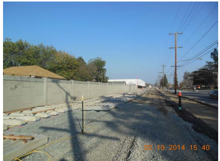
Segment 3: Placing Ties Between Buena Vista and Highland
