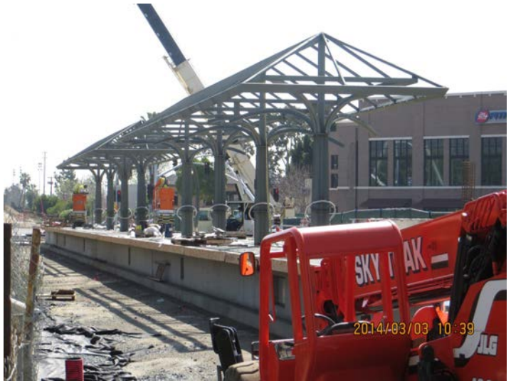
Segment 2: Arcadia Station Canopy Erection
