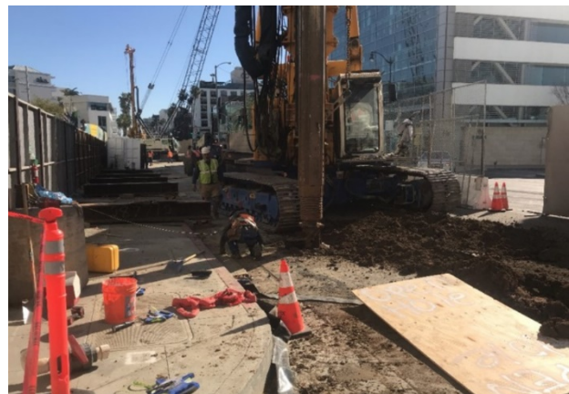
Wilshire/Rodeo Station Pile Installation on Wilshire Boulevard
