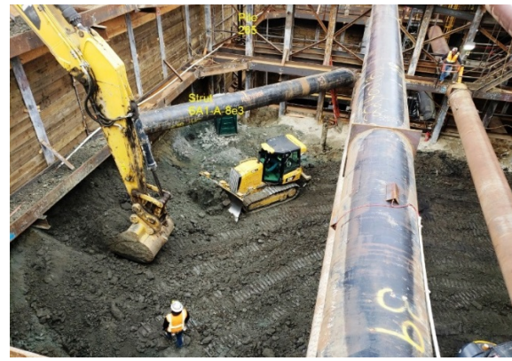
Entrance Appendage Excavation at Wilshire/Fairfax Station
