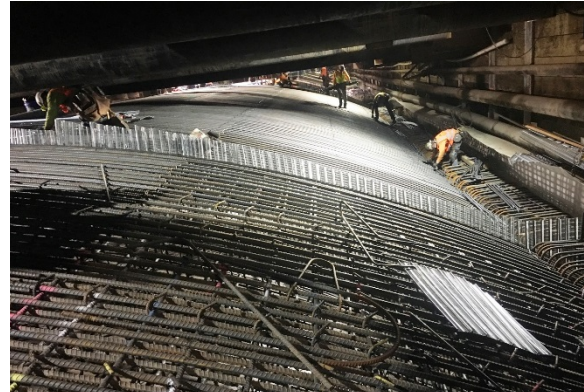
Roof Rebar Installation at Wilshire/La Brea Station
