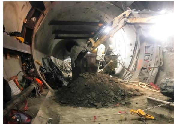
Reach 1 Cross Passage #12 Excavation
