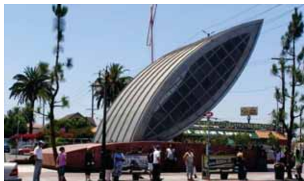
Figure S-51 Entrance canopy at Vermont/ Santa Monica station
