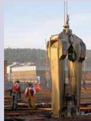
Slurry Wall Excavation, Portland, OR
