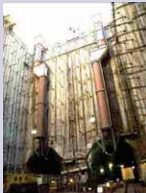
Secant Pile Walls, Barnsdall Shaft, Hollywood
