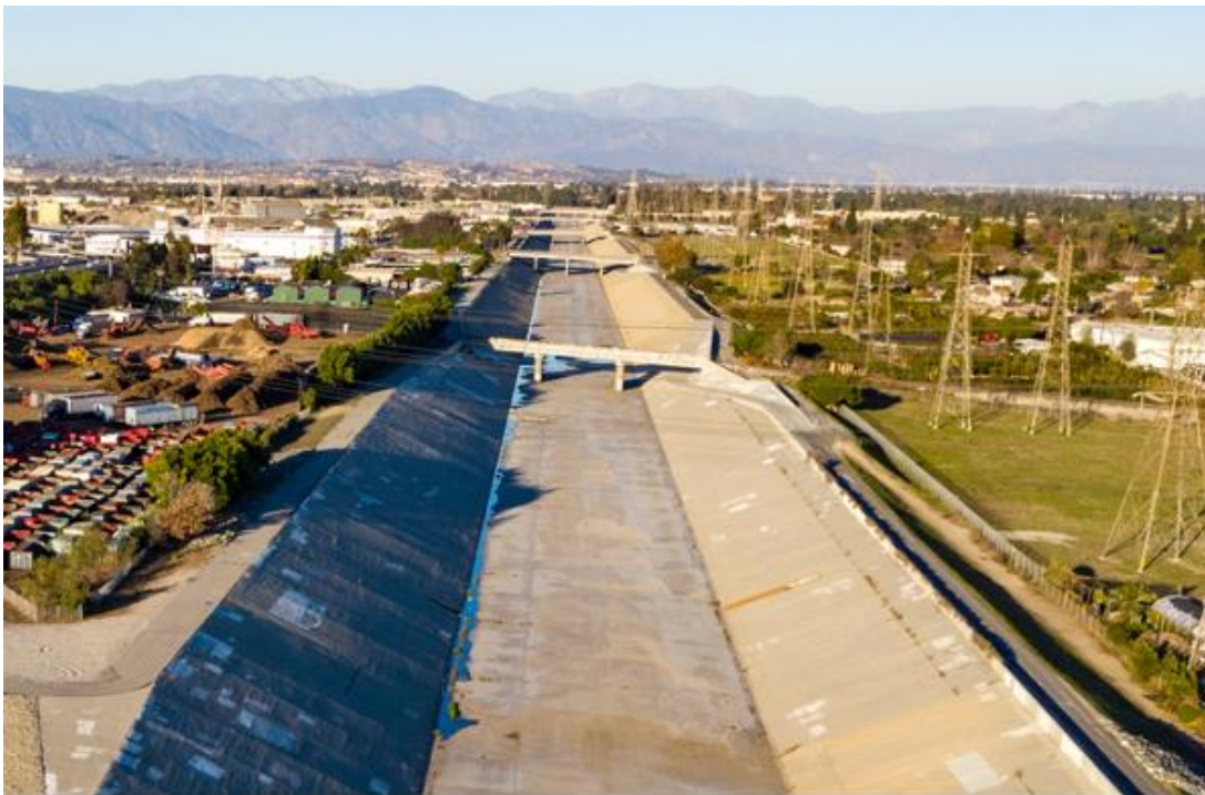
Figure ES 1 Aerial View Looking North Towards the Confluence Station Area
