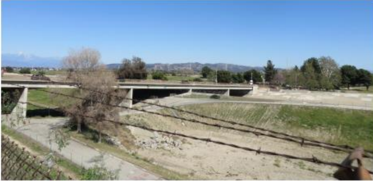
Figure 3.1.14. Viewpoint 13: Washington Boulevard Over Rio Hondo (Looking northeast from Bluff Road)
