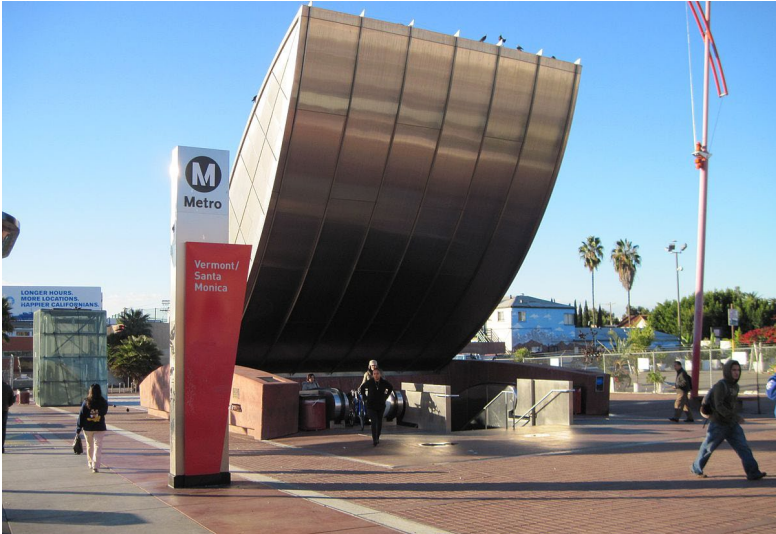
Vermont/Santa Monica Station
