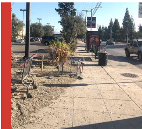
Gravel in sloped planter migrates onto sidewalk, which could obstruct wheeled modes of transportation near station
