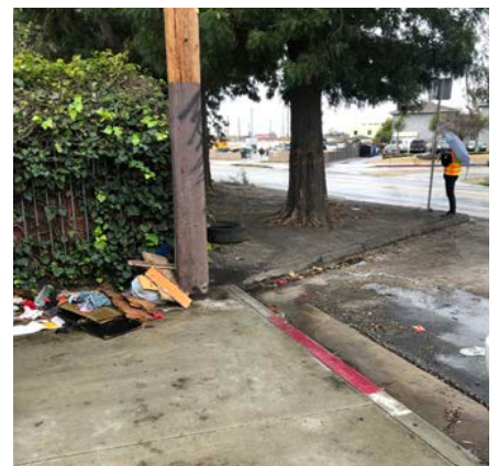
Missing sidewalk and trees planted in center of pathway
