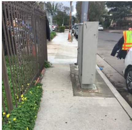
Narrow sidewalk at utility boxes
