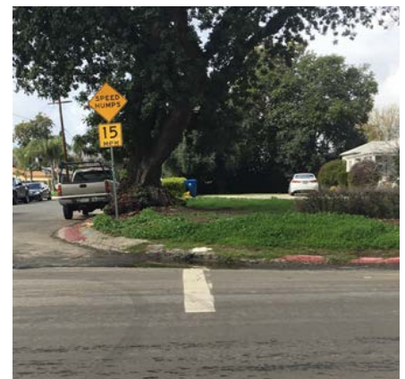
Missing ADA access ramps/sidewalks are unnavigable for anyone
