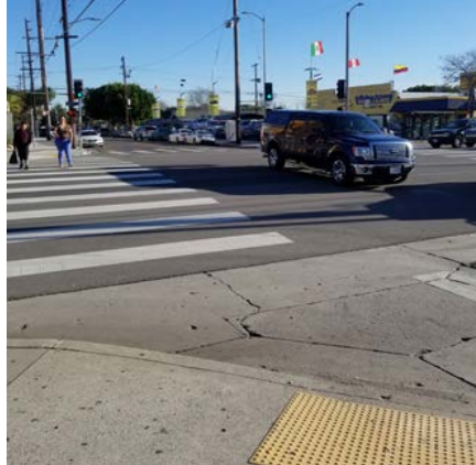
Clear accessible continental crosswalks along Van Nuys Blvd
