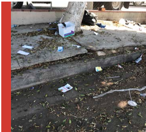
Inaccessible sidewalk due to uplifted pavement and excessive litter
