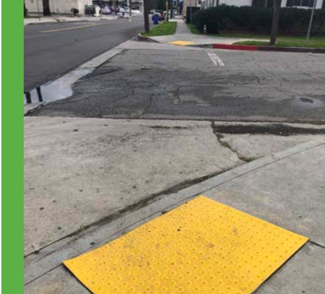
Access ramps with truncated domes seen on secondary pathway intersections
