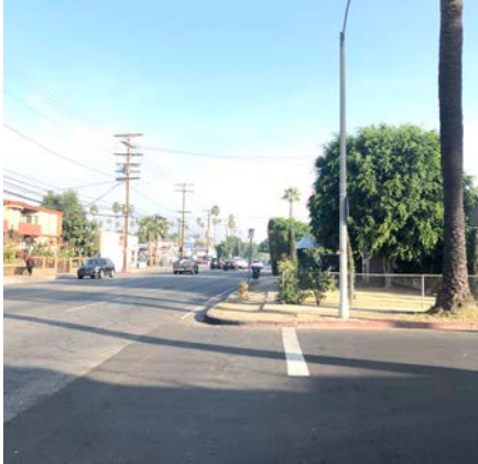
ADA access ramps missing at some corners
