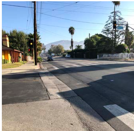
Two clearly marked crosswalks but one missing crosswalk
