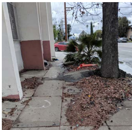
Overgrown palms obstructing sidewalk
