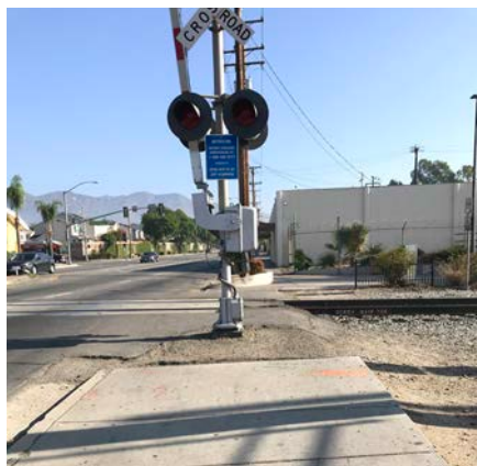
Challenging crossing at rail tracks and uneven crossing of street
