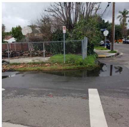
Missing sidewalks in residential area
