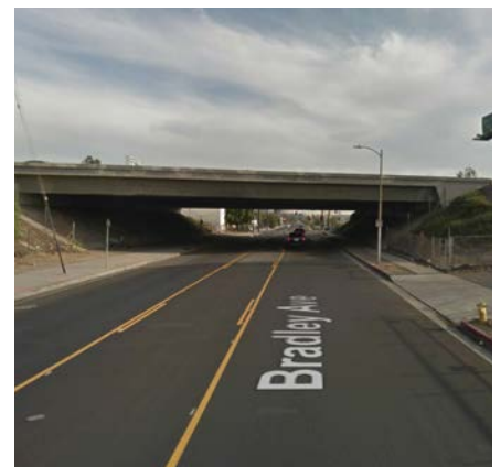
No pedestrian lighting, dark freeway underpass, no eyes on the street
