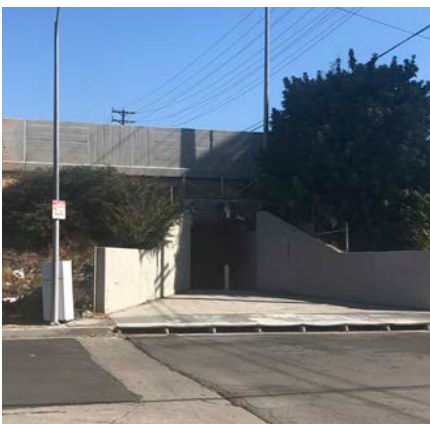
Pedestrian paths at freeway tunnels are dark, narrow and uninviting
