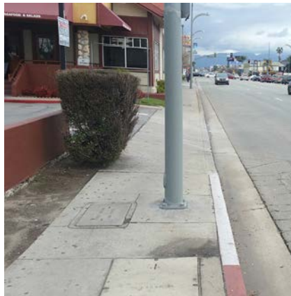
Narrow sidewalks are further constrained by street light poles on Van Nuys Blvd
