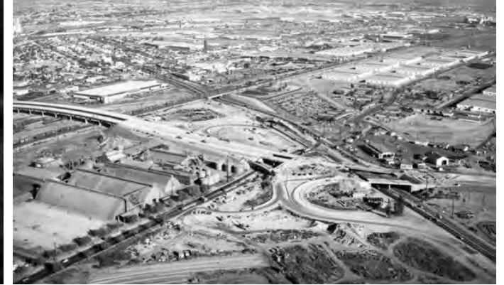
Central Manufacturing District with I-710 under construction in foreground, 1956 (source: Kelly-Holiday Collection of Negatives and Photographs, Los Angeles Public Library)
