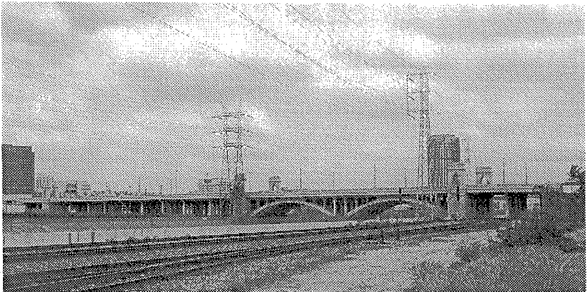
1st Street Viaduct, looking northwest.
