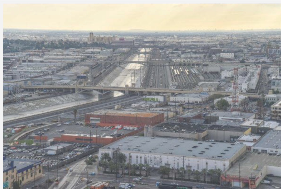
A view of the rail yards for the Red/Purple Line subway and the entrance to the tunnel at bottom left. Photo by Steve Hymon/Metro.
