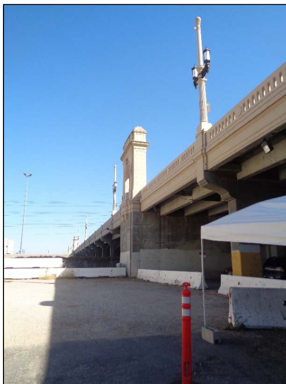
Figure 3.3.1 View of the 1 st Street Bridge from Center Street
