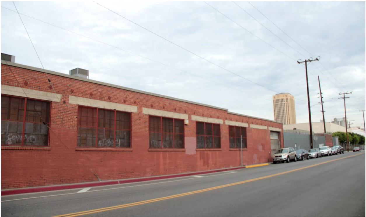
Figure 3.1.10 View Across Center Street from the National Cold Storage Facility
