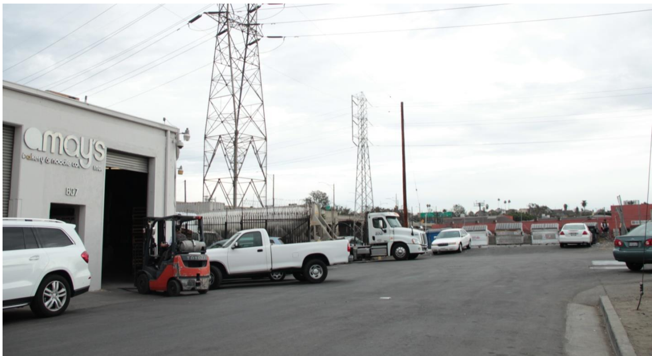
Figure 3.1.3 View of Commercial Street Cul-de-Sac
