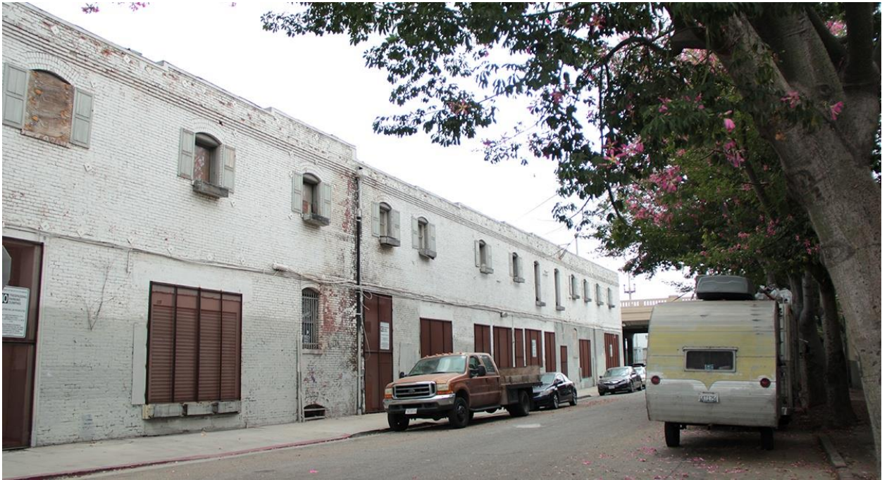
Figure 3.1.12 View of the Citizens Warehouse/Lysle Storage Company Building from Center Street
