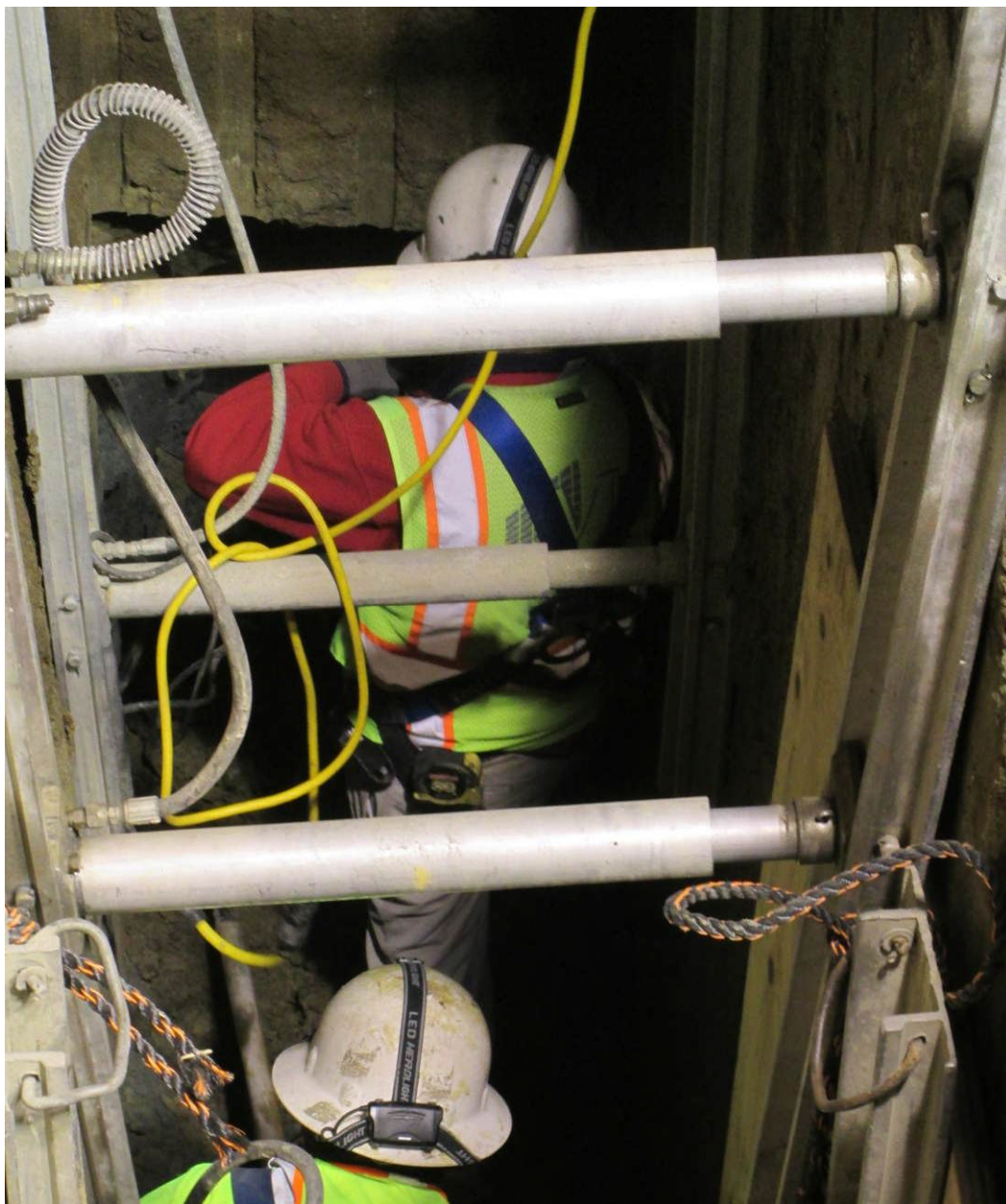
Utility Trench Hand Excavation by the C1048 (Wilshire/La Brea) Contractor.
