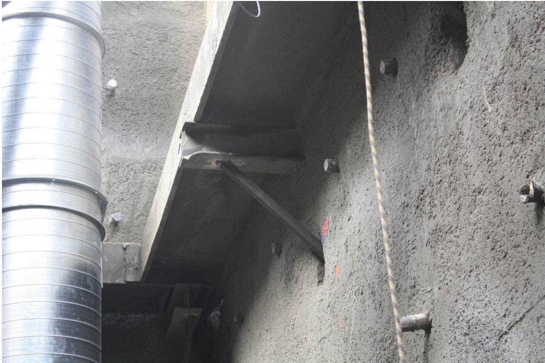
Exploratory Shaft Placement of the First Waler at 15' Level.
